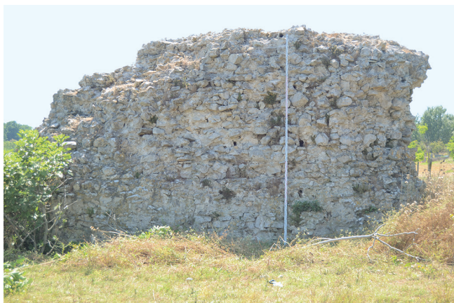
16 a Wall no. 2, east side
