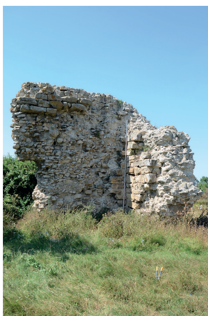
18 a Wall no. 5, east side
