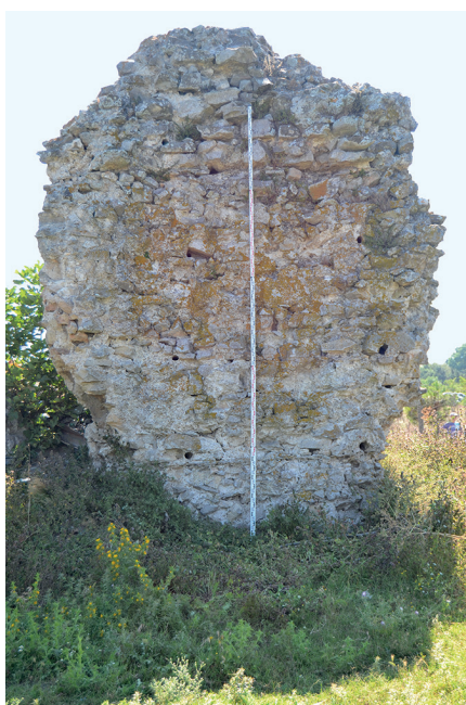
17 Wall no. 4, rows of cut stones
