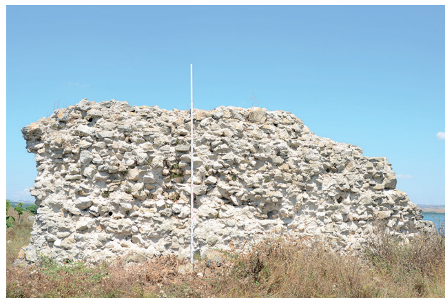
16 b Wall no. 2, west side
