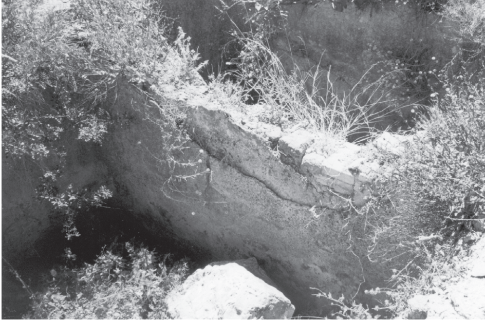
Fig. 19. Cetariae construction: opus signinum facing over rubble construction, visible at Cotta (photo: A. Trakadas).
