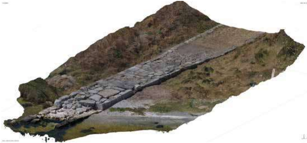
Şek. 6: İskelenin fotogrametrisi (Fotoğraf: Y. Dellal) Fig. 6: Photogrammetry of the jetty (Photograph: Y. Dellal)
