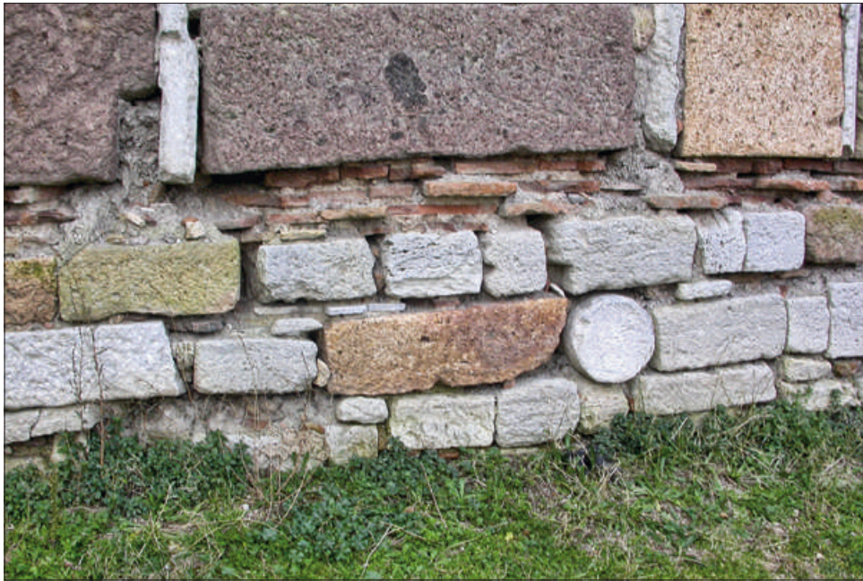
Fig. 7 Ainos. Detail of a wall section of the Byzantine castle. – (Photo Th. Schmidts).
