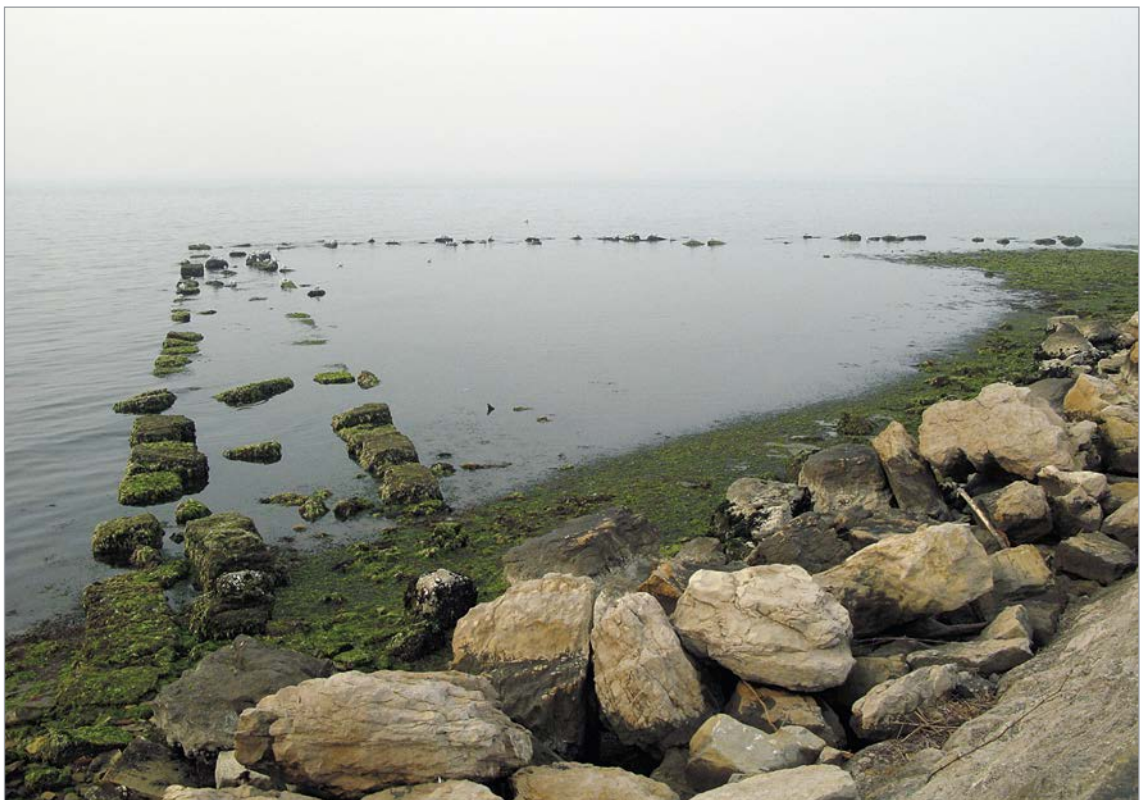
Fig. 14. Roman port structure at Viližan, 23 Feb 2008, 16.00 hours, 65 cm below mean sea-level (photograph: Andrej Gaspari).
