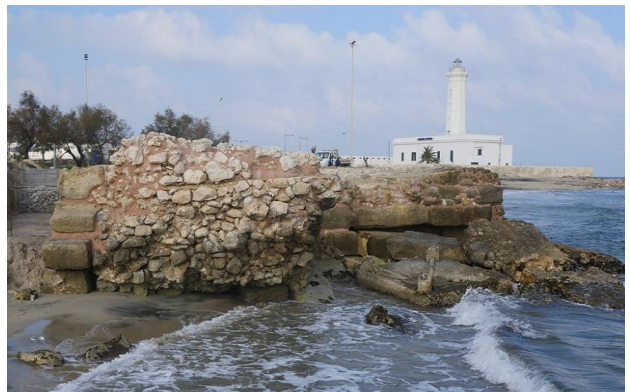
Figure 11: The southern end of pier with opus caementicium (Roman concrete) between the curtain walls in opus quadratum (squared blocks).
