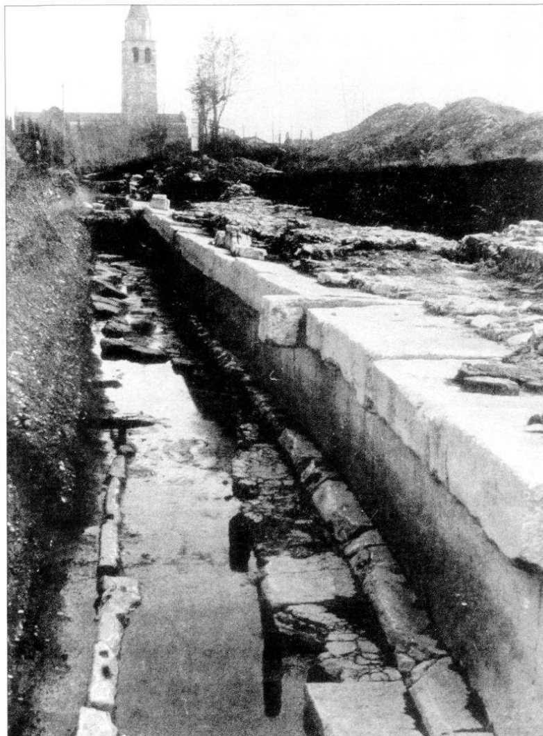
Photo 1 – Portion of the quay discovered along the Roman fluvial harbour of Aquileia (photo by G. Brusin). The structure is situated on the right bank of the Natissa palaeochannel.
