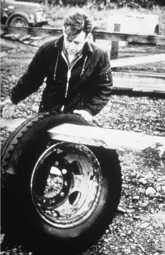
Photo of objects broken by force of wave—plank was forced through the tire during 1964 earthquake-related tsunami in Alaska (USGS)
