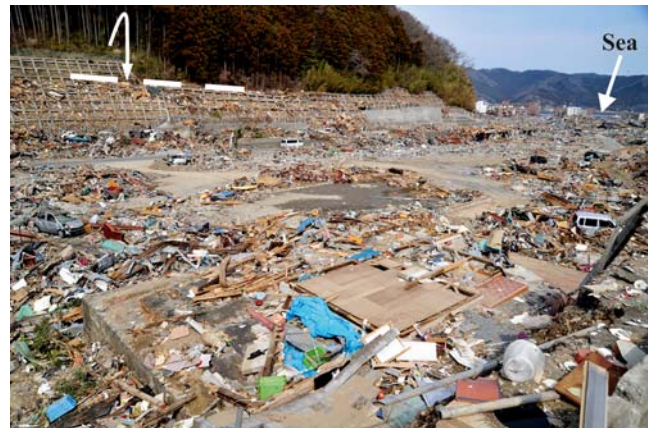
Figure 3. Estimation of run-up approximately 28 m (tsunami flow depth > 10 m), in the area of Onagawa (Japan, 2011). The area has been totally destroyed and intensity values reached XII ITIS-2012 . The color version of this figure is available only in the electronic edition.
