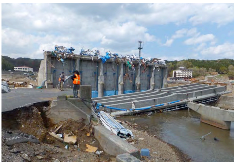
Figure V-4: Field survey of Iwate Prefecture Japan. Georeferenced Photo label is: DSCF0248_5-13-11_Taro Fishing Port_Bridge Deck System Turned Upside Down off Piers Adjacent to Canal Control Structure_RMN.JPG
