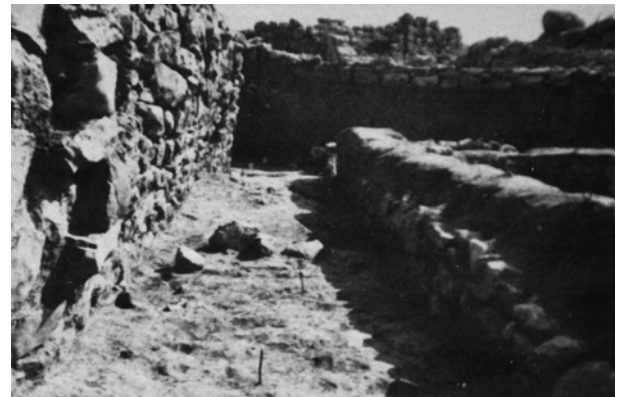
Figure 15. Tilted eastern and western walls within Building VI at Tiryns (after Kilian, 1996: fig. 5).
