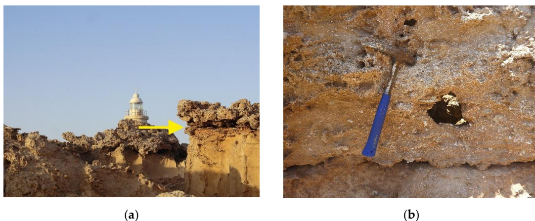
Figure 10. (a) The subaerially eroded red horizon that has acted as a detachment zone is indicated by a yellow arrow; (b) detailed view of this detachment zone.
