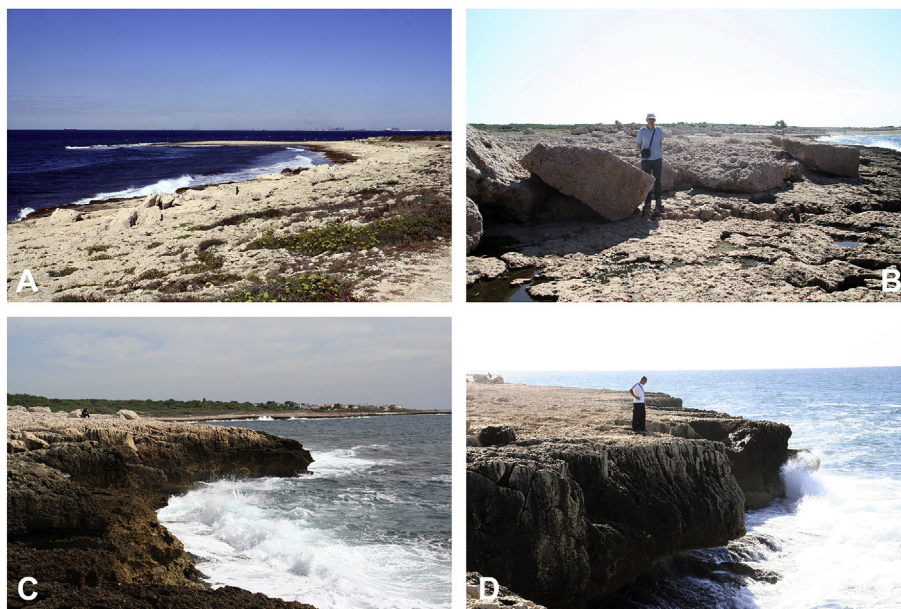
Fig. 4. Morphological features of the studied area. A: gently sloping rocky coast characterized by boulder accumulation and soil cover; B: boulder field in the surveyed area; C: cliff about 4 m high; D: notch at the foot of the cliff.
