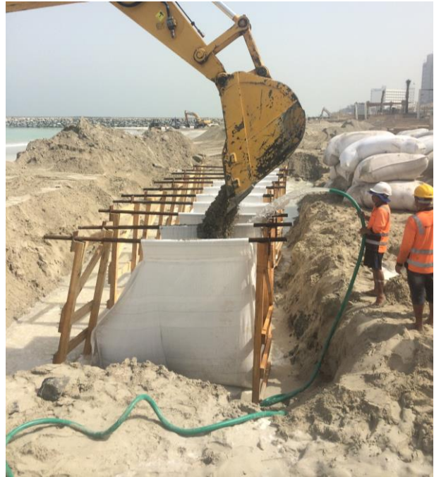
Figure 8 Filling “Trapbags” containers as freestanding core
