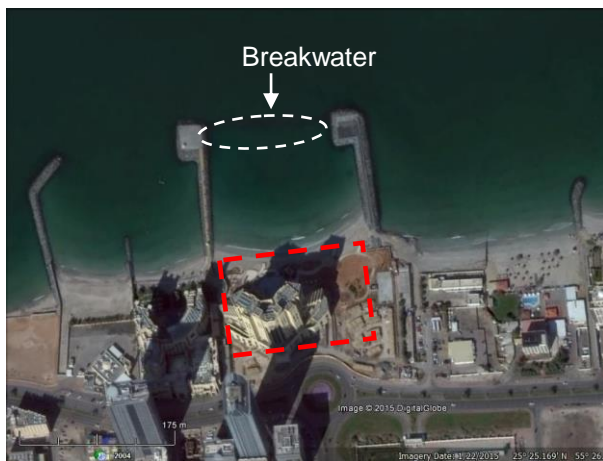
Figure 1 Site with existing groynes and low crested submerged breakwater
