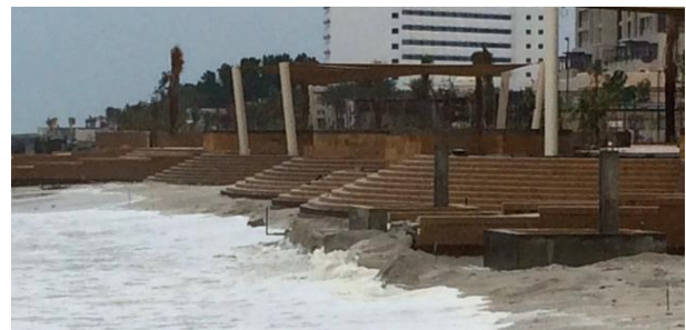
Figure 2 Storm (shamal) wave in January 2015 eroding recently nourished beach up to hard landscaping.
