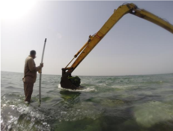
Figure 7 Placing 3-6t armour rock tightly at low tide
