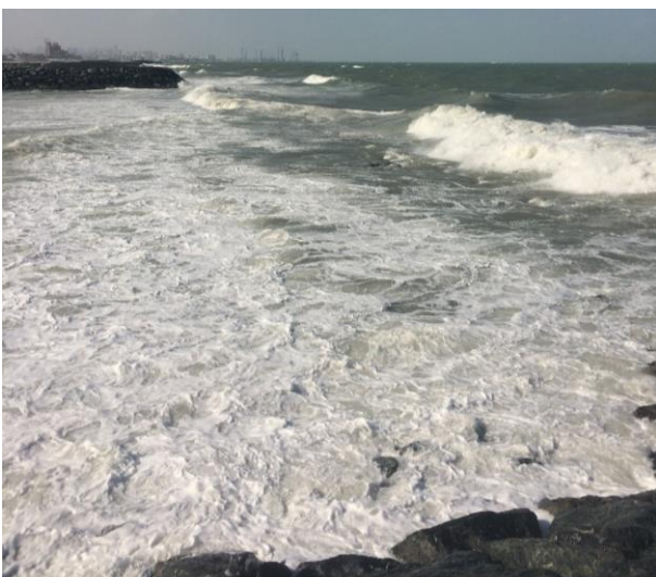
Figure 11 Photo of performance of submerged breakwater during mid-tide (0.9m LAT) with wave breaking ( H_s \sim 1.5m )
