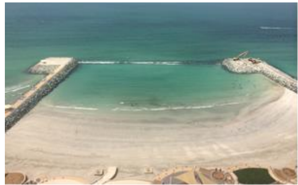
Figure 13 Completed works with waves breaking on breakwater and terminal wall buried under nourished beach.
