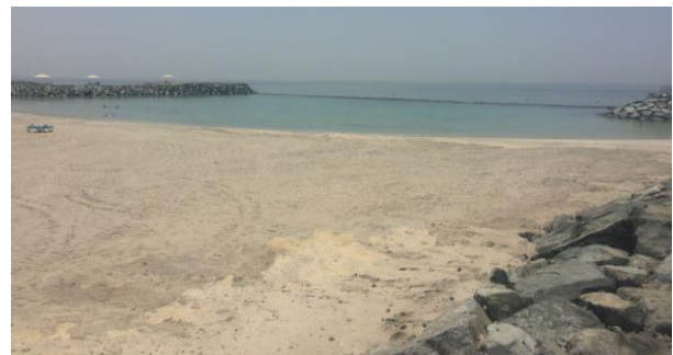
Figure 14 Wide stable beach at low tide, submerged breakwater visible through water on clear day
