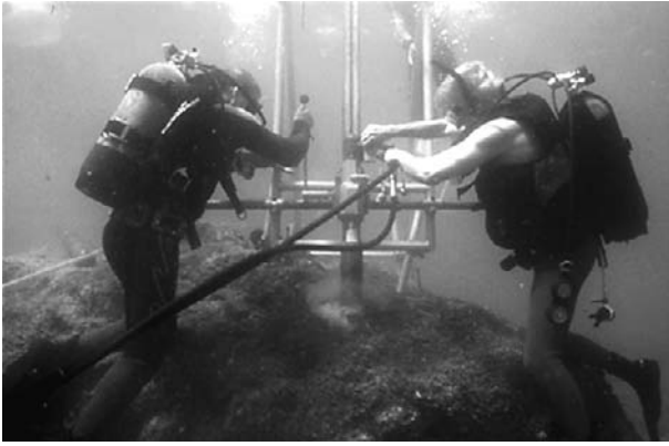
PHOTO 2 - ROMACONS CORING RIG WORKING UNDERWATER (Cliché : R.L.HOHLFELDER, 2003)
