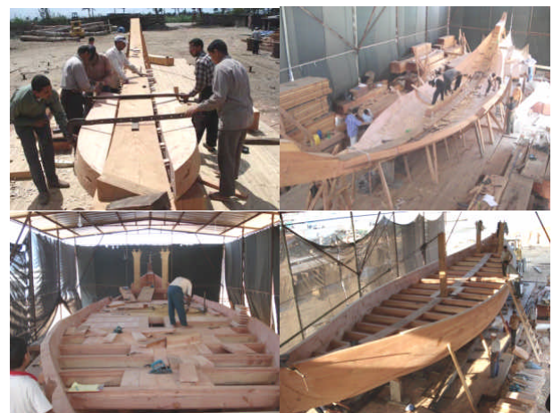
Figure 18: Min at various stages of construction
