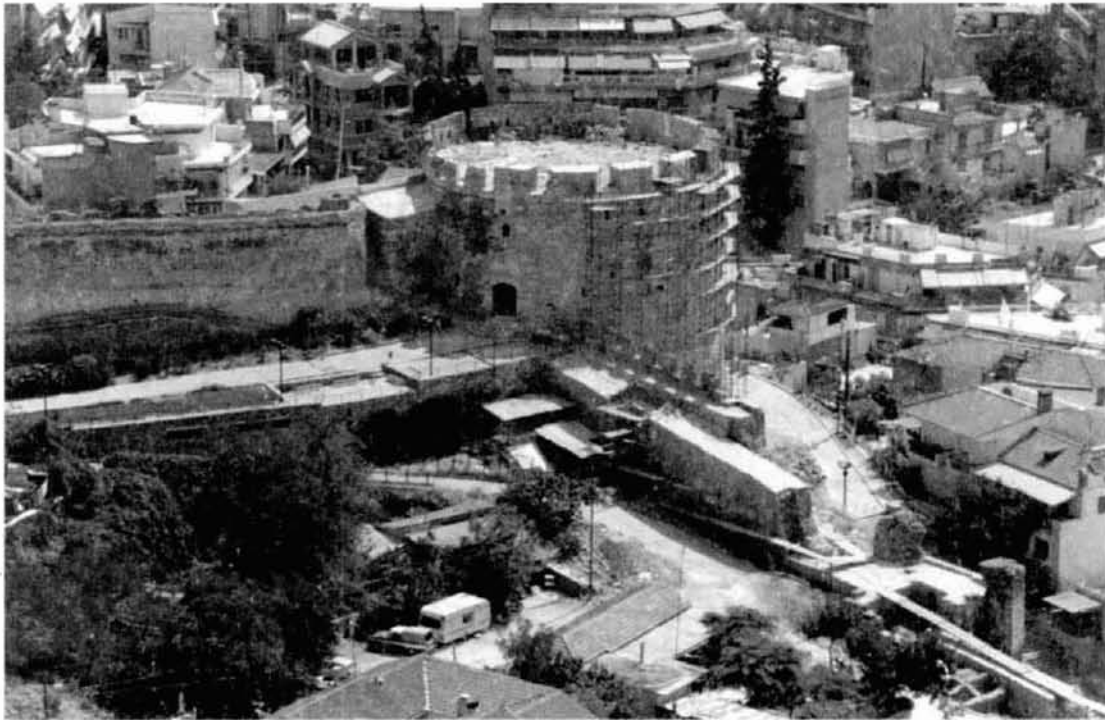
The Trigonian Tower with the excavation area and the cisterns protected by roofing
