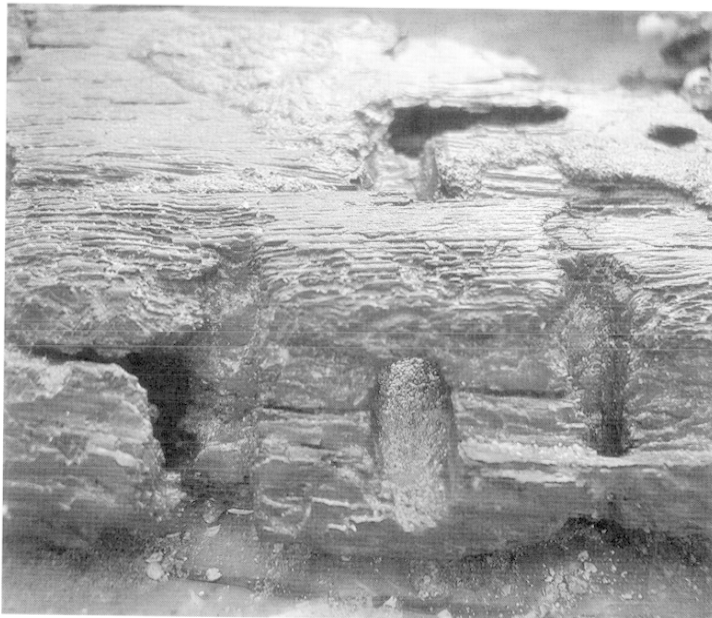
Fig. 5 : Repair dowel hole in fragment UM3. (Photo M. Polzer).
