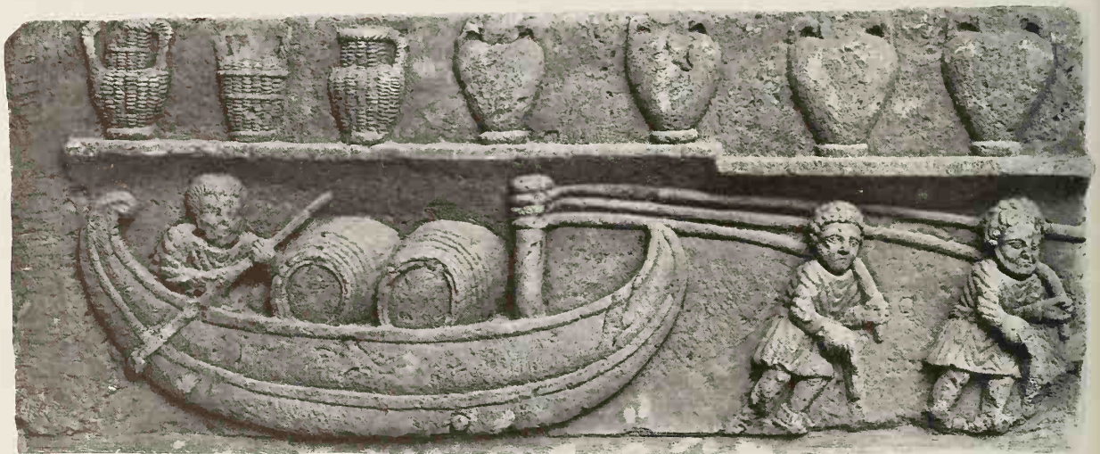
97 A small rivercraft being hauled by a towline made fast to the top of the towing mast. On larger rivercraft the line would pass over a block on the mast and be made fast to a capstan near the stern. Relief found at Cabrières-d'Aigues and now in the Musée Calvet, Avignon; 3rd century AD.
