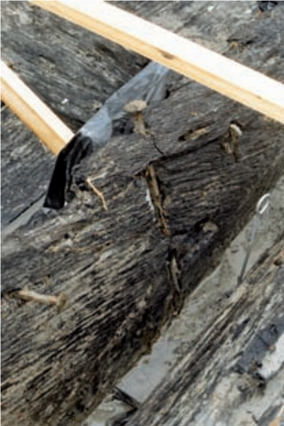
Fig. 2. Long nail running through scarf between two elements of the L-shaped chine (photo T. Penders, RCE).
