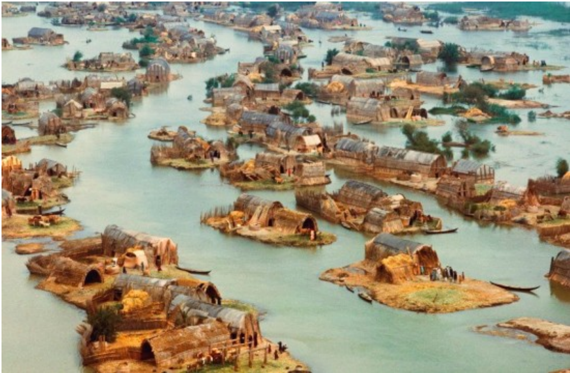
Figure 40: Raft: Typical mudhif floating basket homes or rafts or reed islands are traditional housing in Ma'dan in River Tigris catchment area in Iraq. It is not unique in the world while similar tradition is also recorded on Titicaca Lake in Peru as well as Aztec tradition of both housing and gardening on floating reed rafts big enough to be called floating islands. (Photography: Vanessa MessyNessy [On line] Available at: < http://www.messynessychic.com/2014/11/12/the-floating-basket-homes-of-iraq-a-paradise-almost-lost-to-saddam/ > [29. May 2015]).
