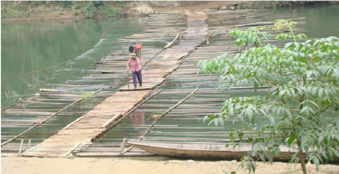
Figure 57: Some special forms of using water and possibility of floating, which could not be understood as navigation, but is in any way important for migration. These can also be the matter of different kind of early floating bridges. Bamboo floating bridge on River Xam near Xam Tai in jungle of Nam Xam Nature Reserve in western Houaphon in Laos (Photography: Josh Hirschstein ©Travel Ventures [On line] Available at: < http://hilltribeart.com/wordpress/?p=406 > [29. May 2015]).
