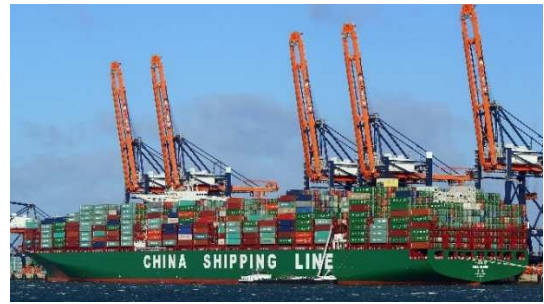
Five gantry cranes with arms lifted allowing ship movement. A berth of this type can move around 150 TEU per hour (picture https://www.marinetraffic.com ).
