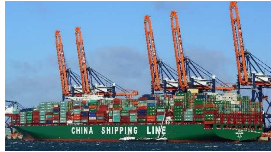
Five gantry cranes with arms lifted allowing ship movement. A berth of this type can move around 150 TEU per hour (picture https://www.marinetraffic.com ).
