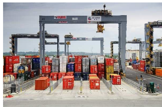
Fully automated container park at the London Gateway (picture http://www.kalmar.fr ).
