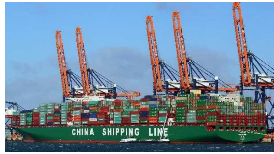
Five gantry cranes with lifted arm allowing ship movement. Such a berth can move around 150 TEU per hour (picture https://www.marinetraffic.com ).
