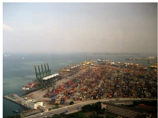
Singapore's container terminals total nearly 60 berths on 17 km of quay, over 200 gantry cranes and large areas for container storage (Wikipedia).
