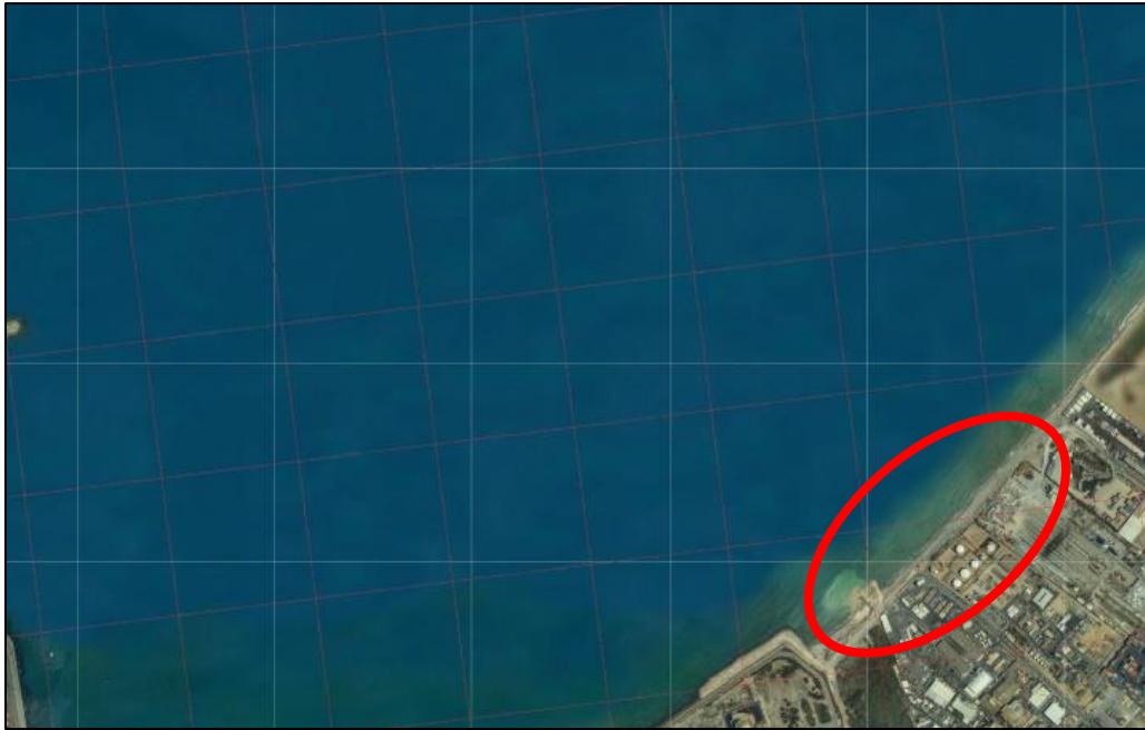
Figure 23: Starting the construction of the new Lee Breakwater (June 2015)
