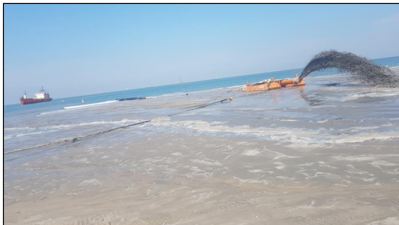
Figure 26: Trailer suction hopper dredger pumping sand ashore
