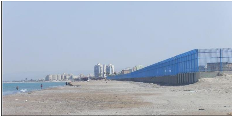
Figure 28: Beach width in front of concrete fence after sand nourishment
