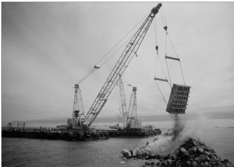
Figure 9.18 Placing armourstone from floating barge using a rock tray/skip (courtesy CUR)
