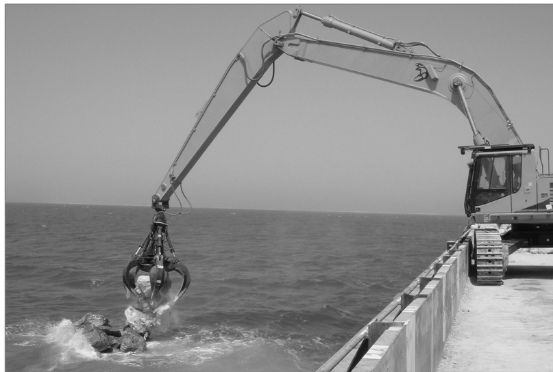
Figure 9.22 Placing armourstone with an excavator (courtesy Van Oord)
