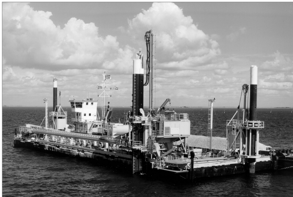
Figure 9.25 Multi-purpose pontoon Scradeway with scrapper installation (courtesy Royal Boskalis Westminster)
