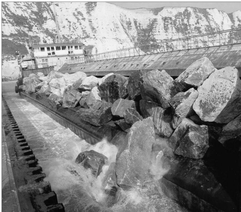
Figure 9.21 Side stone-dumping vessel Cetus dumping 1–3 t armourstone near a jetty (courtesy Royal Boskalis Westminster)
