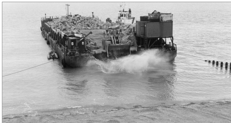
Figure 9.13 Wheel loader working from beached barge (Royal Boskalis Westminster)
