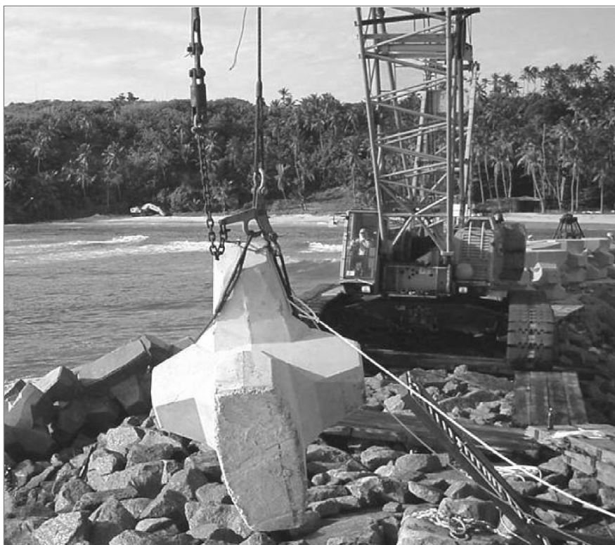
Figure 9.61 Use of a quick-release hook (courtesy Interbeton)
