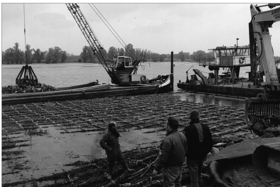
Figure 9.67 Fascine mattress in position, beginning of ballasting (courtesy Van Oord)
