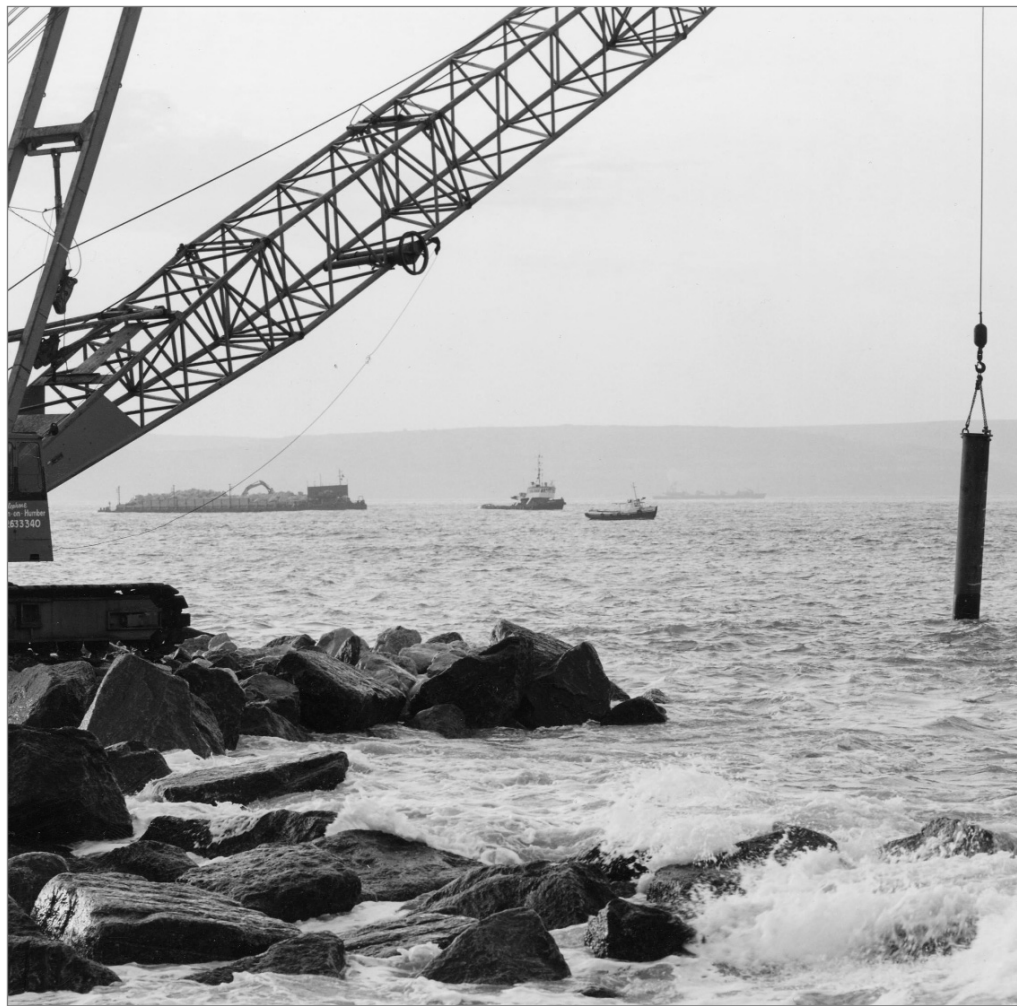
Figure 9.70 Underwater profile checks with a sounding rod (courtesy David Bowie)
