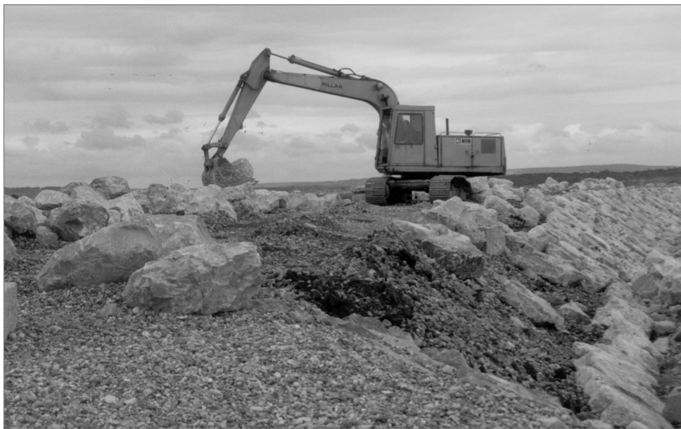
Figure 9.14 Excavator working on the crest (courtesy J D Simm)
