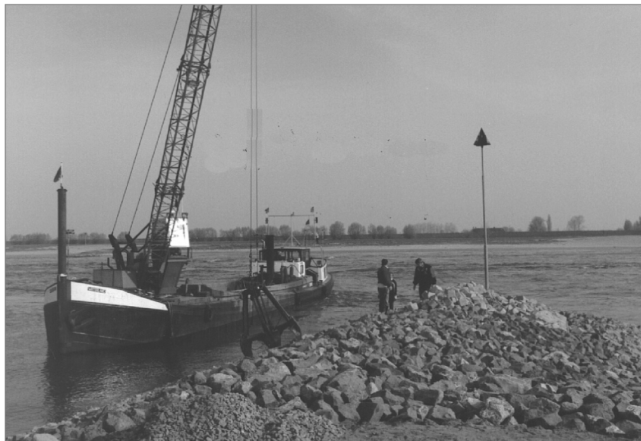
Figure 9.68 Placement and trimming of spur-dike capping layer (courtesy Van Oord)
