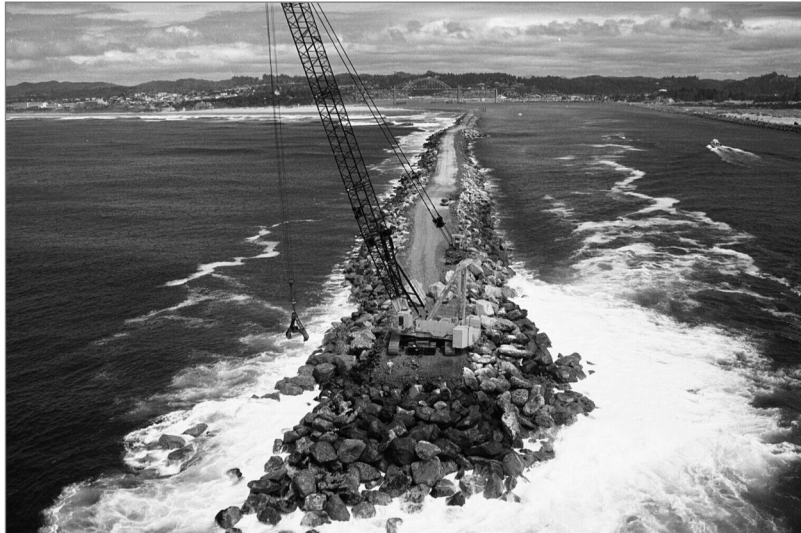
Figure 9.15 Crawler crane working on breakwater crest (courtesy Brien Wegner, USACE)
