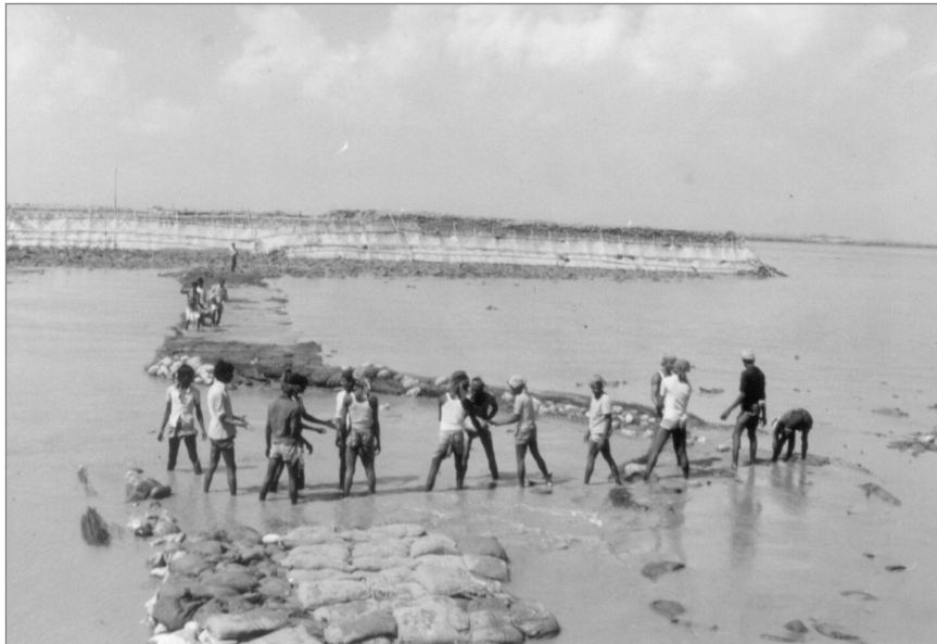
Figure 7.29 Sill in estuary closure, Feni River, Bangladesh (courtesy J van Duivendijk)
