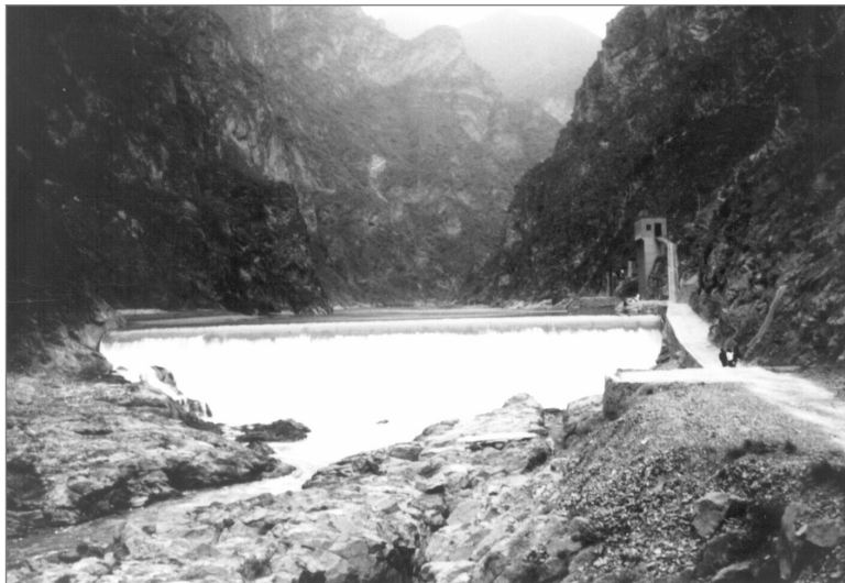
Figure 7.33 Diversion dam in China (downstream face) (courtesy J van Duivendijk)
