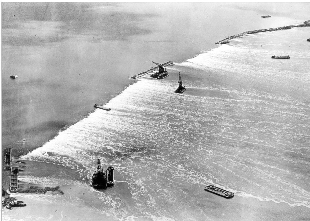
Figure 7.30 Bed protection in Schelphoek shallow closure, the Netherlands (1953) (courtesy KLM)
