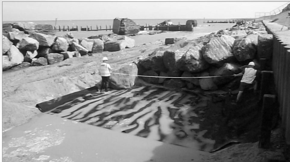
**Figure 6.71** Construction of Corton coast protection scheme, UK (courtesy Halcrow)
