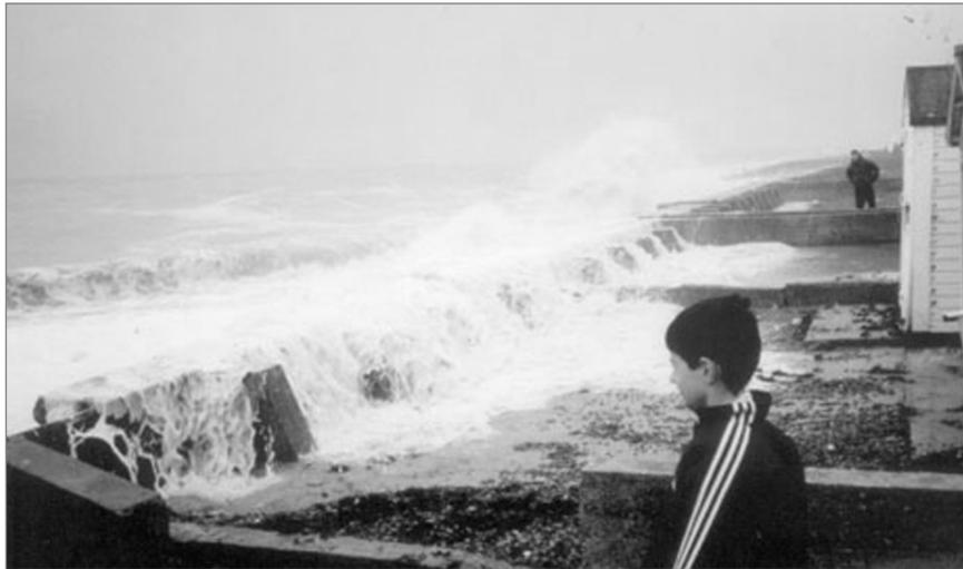
**Figure 6.54** Overtopping of seawall. Note pedestrians and proximity of small buildings (courtesy Halcrow)
