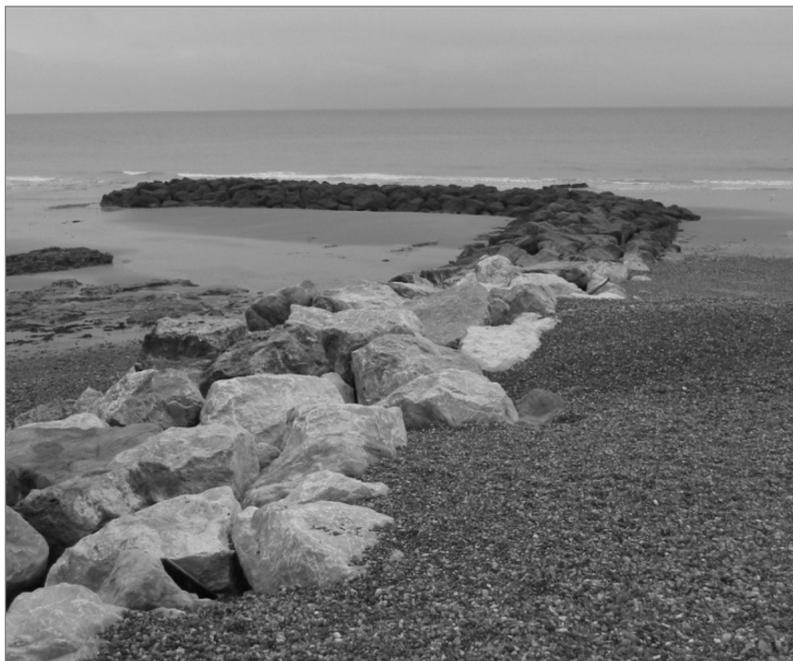
Figure 6.47 L-shaped groyne, Bulverhythe, UK (courtesy Halcrow)
