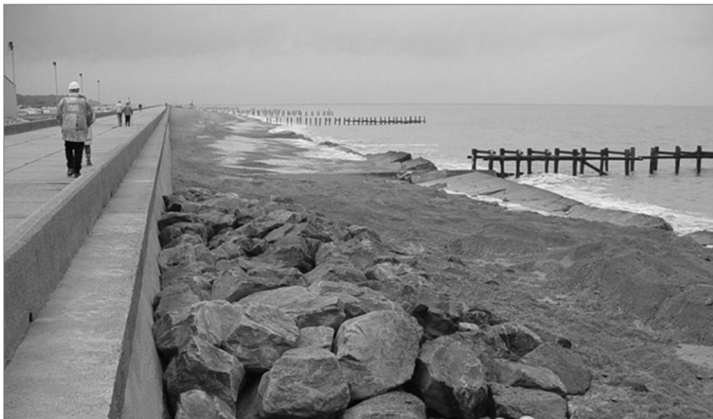
**Figure 6.49** Rock revetment to protect a concrete seawall (courtesy Halcrow)
