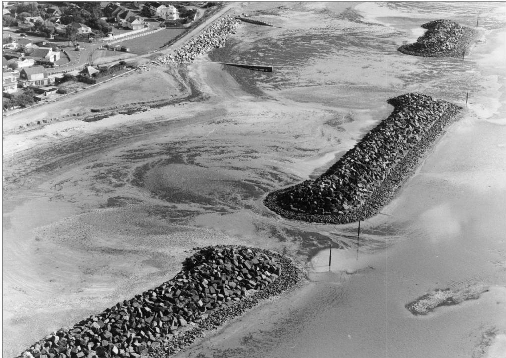
**Figure 6.77** *Detached breakwaters, Elmer, UK (courtesy Environment Agency)*
