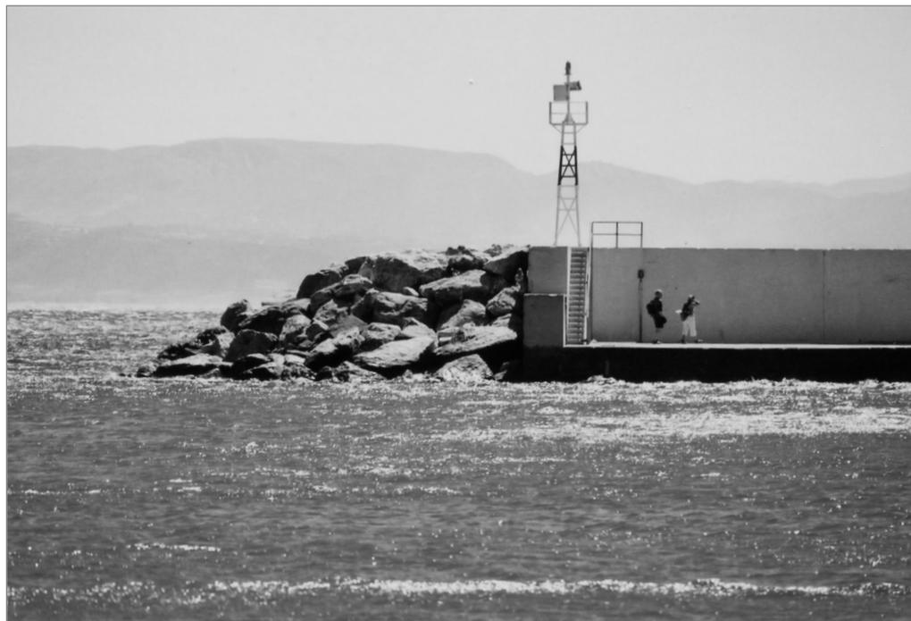
**Figure 6.9** *Armourstone protection on breakwater roundhead, adjacent to vertical caisson (courtesy Clive Orbell Durrant)*
