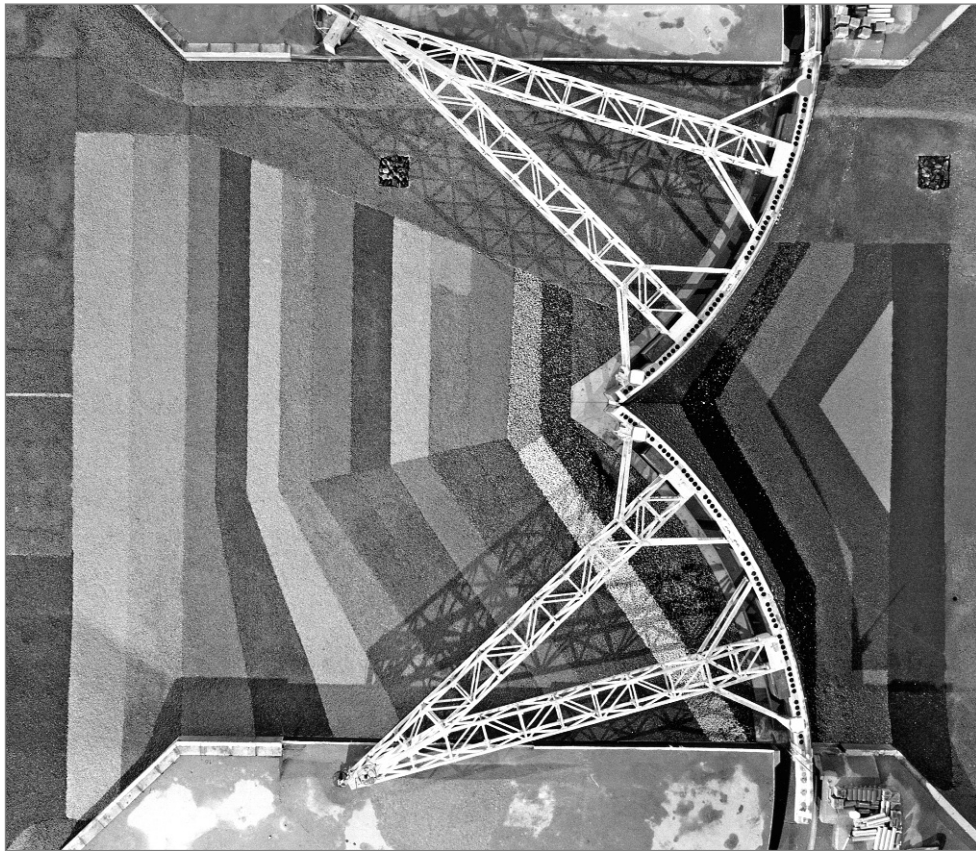
Figure 5.120 Plan view of the set-up for the evaluation of the stability of the bed protection of the Maeslant storm surge barrier in the Netherlands (by WL|Delft Hydraulics for construction consortium Maeslantkering and Rijkswaterstaat)
