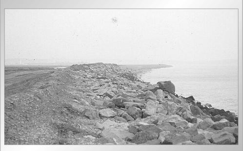
Figure 10.9 Hurst Spit armourstone revetment in December 1989, after storm damage (courtesy A P Bradbury)
