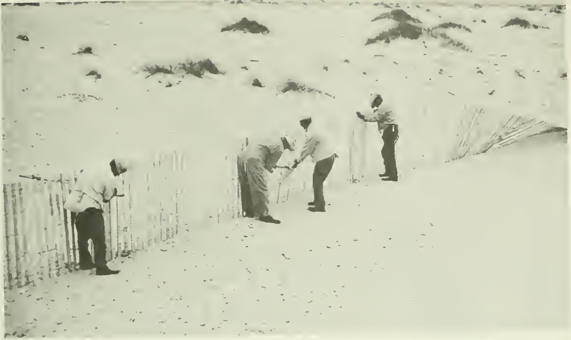
Figure 6-26. Erecting snow-type sand fencing.
