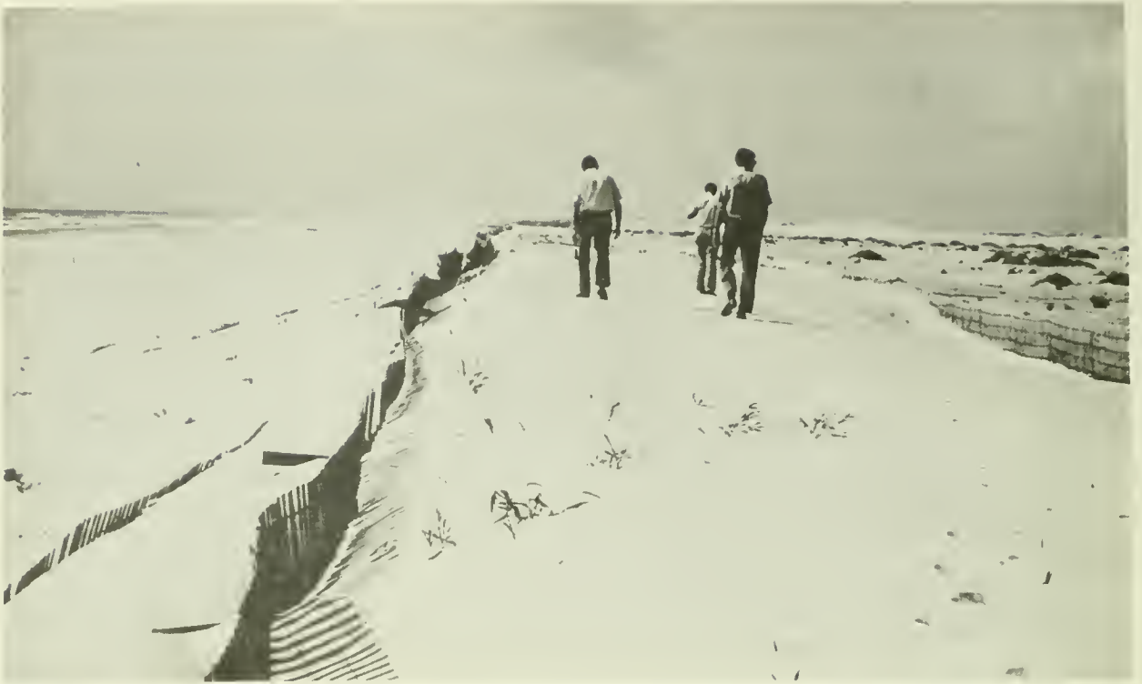
Figure 6-27. Snow-type sand fencing filled to capacity, Padre Island, Texas.
