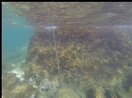
the basement of the lighthouse
