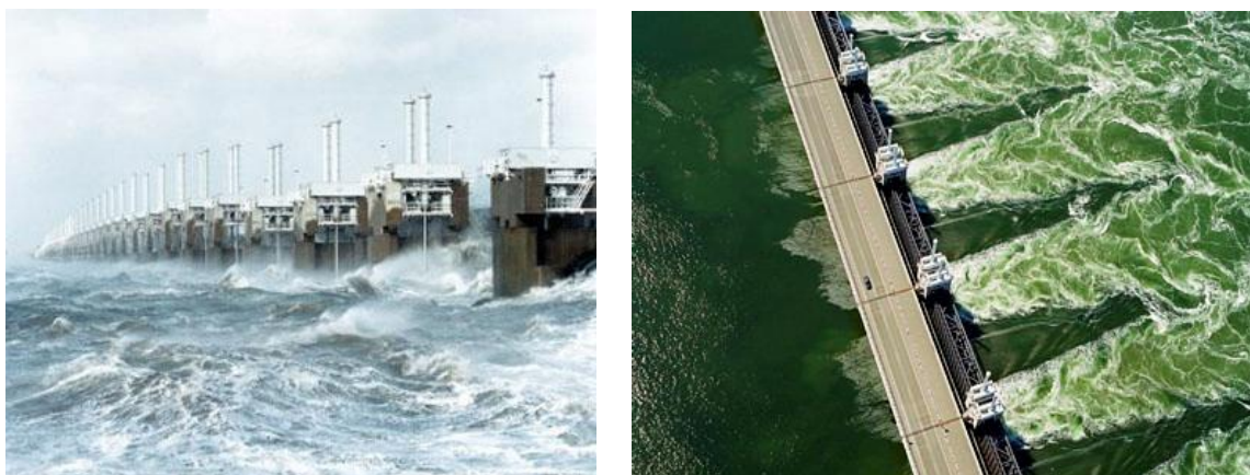
Figuur 1.1 Left: Eastern Scheldt Storm Surge Barrier during a storm and Right: tidal flow through the gates of the Eastern Scheldt Barrier during ebb (© Rijkswaterstaat).
