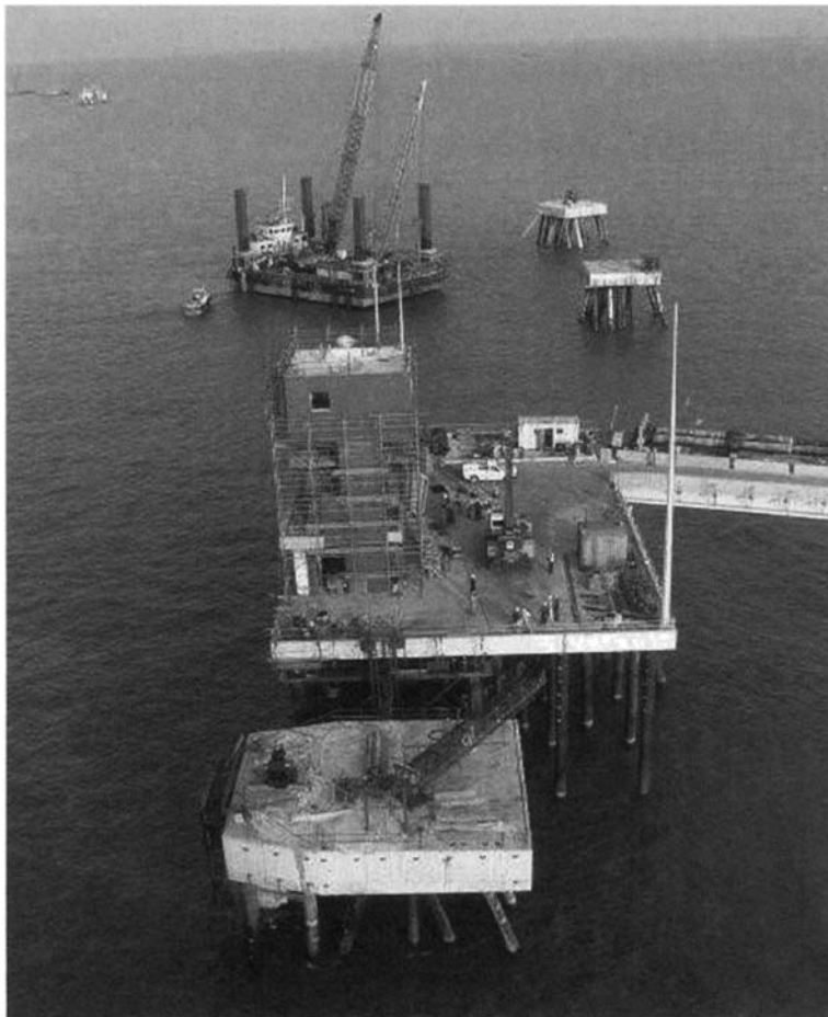
Figure 5.11. Dabhol jetty head under construction (courtesy Besix-Kier)
