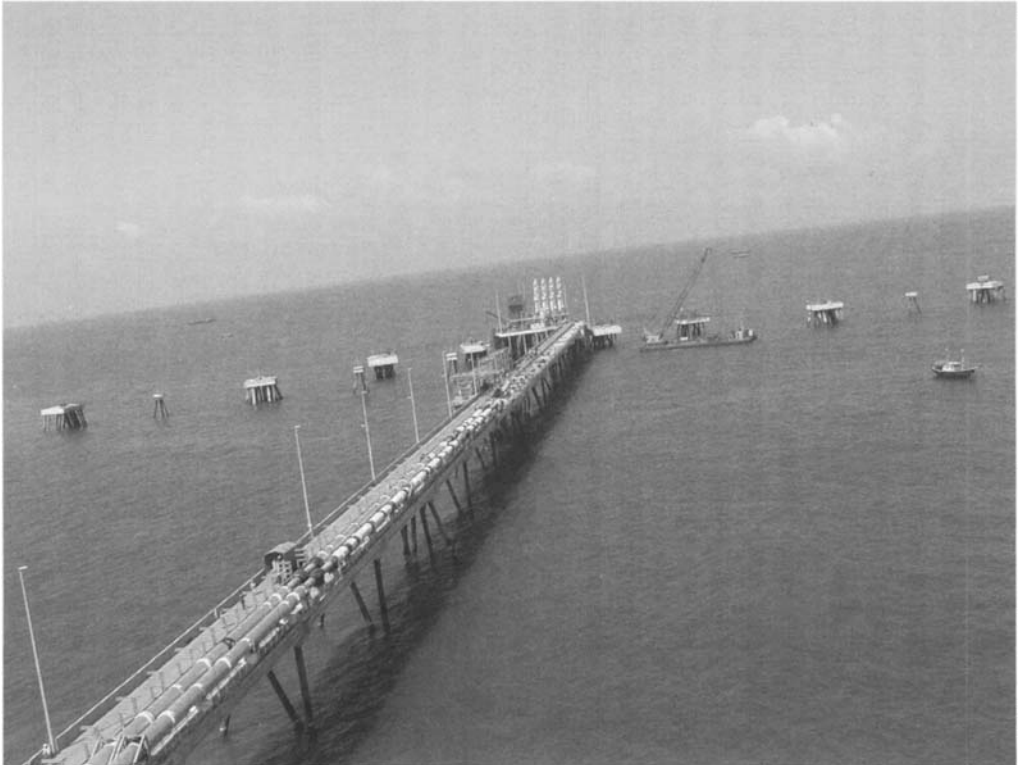
Figure 6.1. Jetty head and mooring dolphins under construction, Dabhol (courtesy Besix-Kier)
