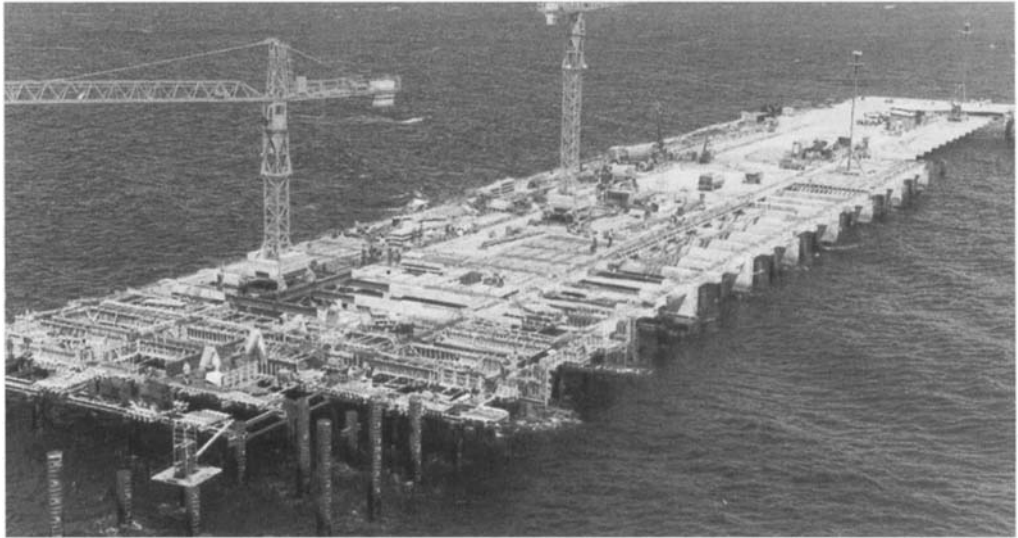
Figure 8.1. Aqaba jetty under construction (courtesy Mott MacDonald and C J Associates)
