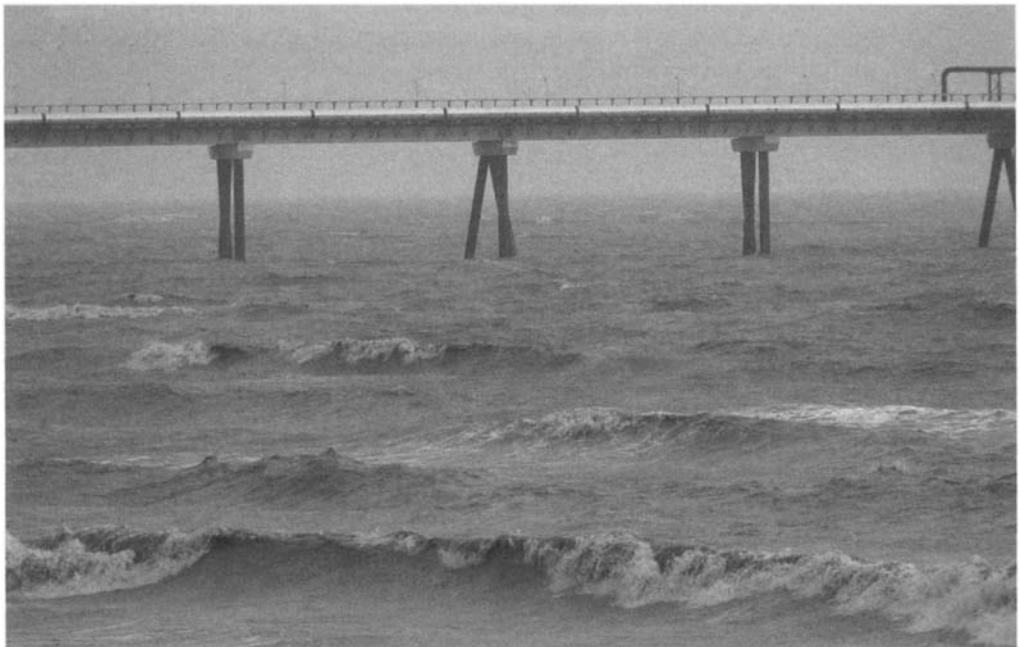
Figure 3.3. Wave breaking in calm conditions (checks should be made to assess whether under extreme conditions waves could break onto the deck section)
