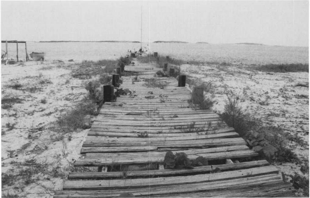
Figure 7.10. Sedimentation can also affect the usability of the jetty! (courtesy Doug Ramsay)
