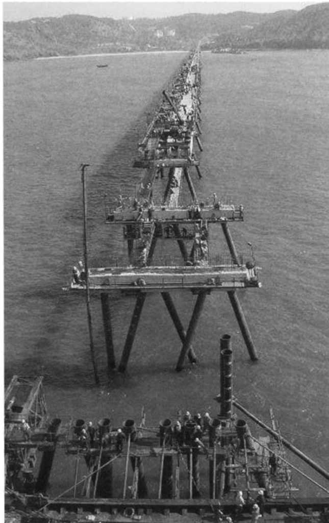
Figure 1.1. Typical exposed jetty under construction (courtesy Besix-Kier)
