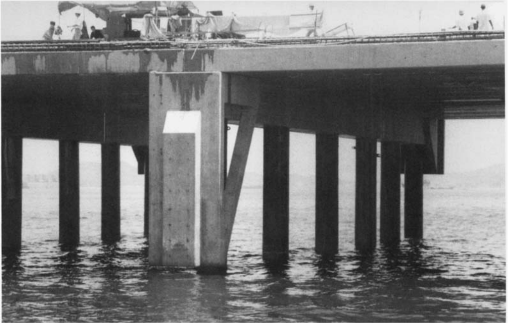
Figure 4.1. Fender panel on an exposed jetty – even when the main structural elements are slender and attract relatively little hydraulic load, additional elements such as fender panels can attract more significant load (courtesy Kier)
