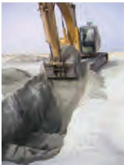
Figure B.18 Excavation of a test pit in hydraulic fill.
