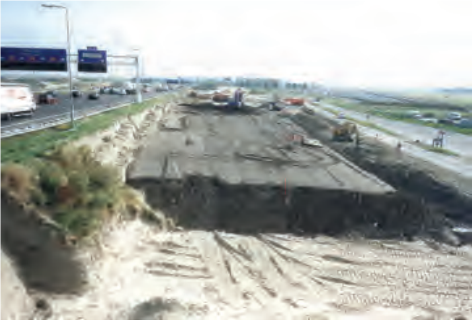
Figure 9.12 Construction of highway exit with dredged (ripened) clay.
