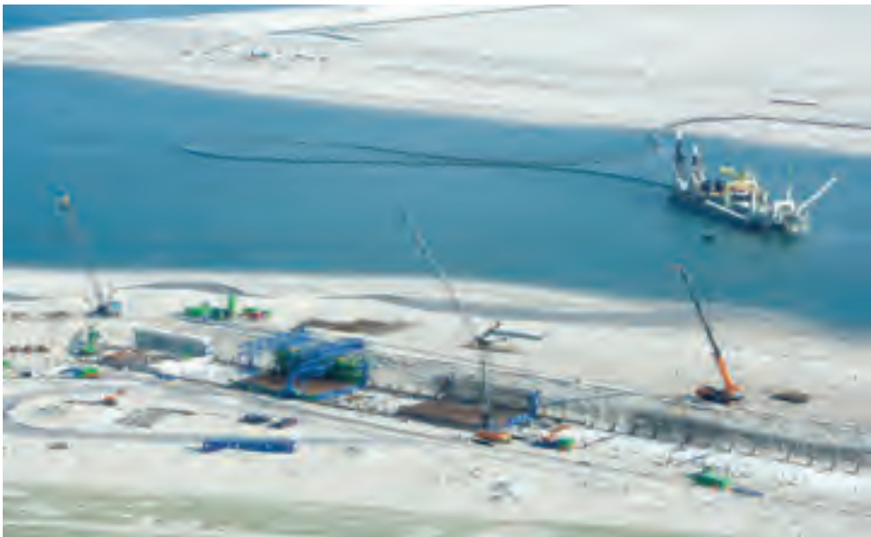
Figure 10.8 Simultaneous dredging and construction works at Maasvlakte 2, Rotterdam, The Netherlands.
