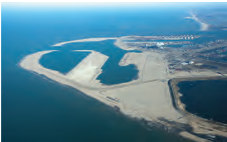
Figure 1.1 Construction of Maasvlakte 2 in progress, Rotterdam Europoort, The Netherlands, October 2011.
