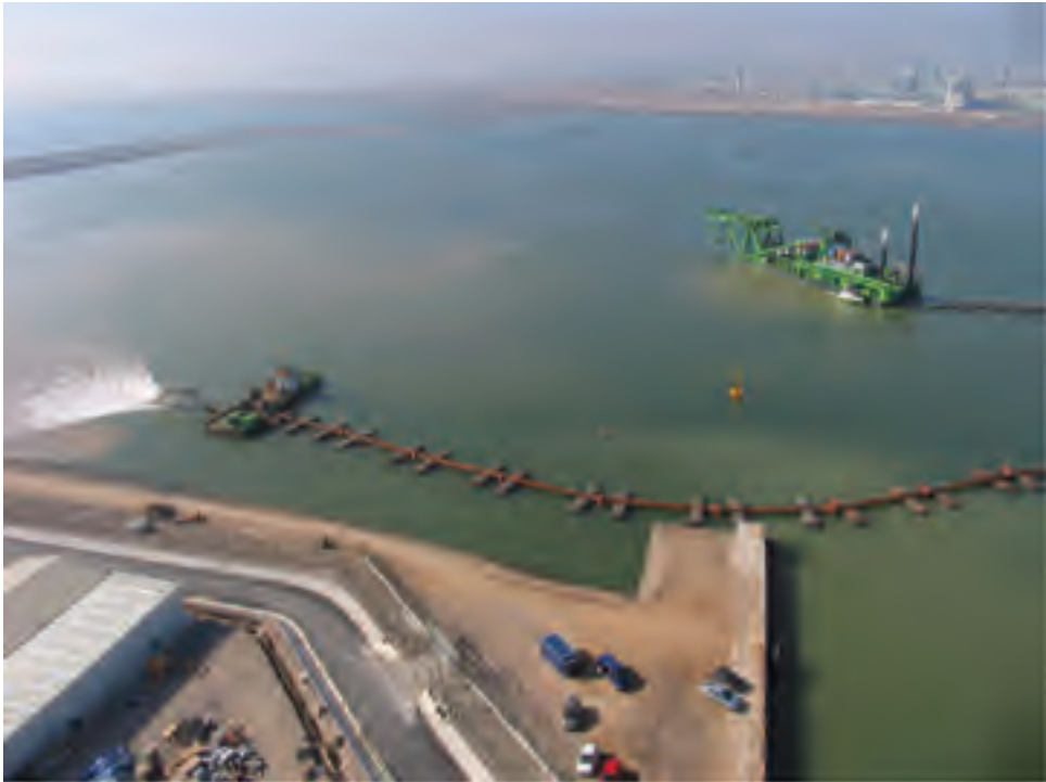
Figure A.33 Floating pipe line on small steel pontoons.
