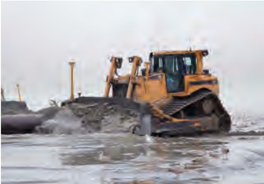
Figure A.42 Distribution of fill material by bulldozer.
