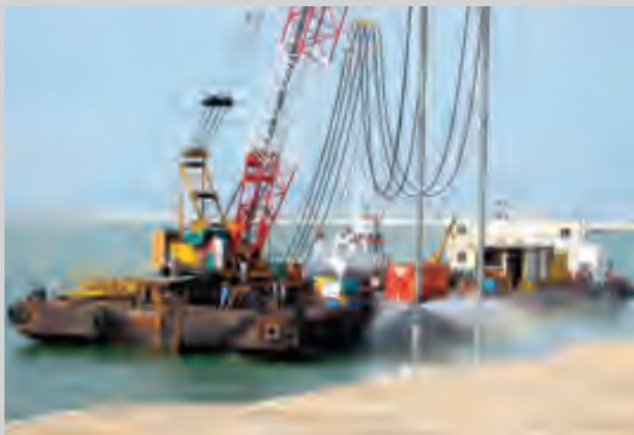
Figure 7.16 Compaction of the slope of a reclamation in Singapore (info Keller).
