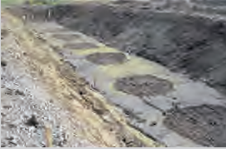
Figure 7.24 Top of dynamic replacement columns after installation and excavation (info Menard).
