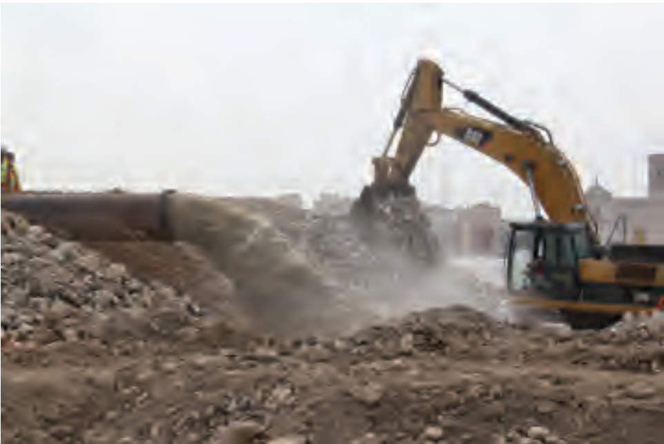
Figure 9.34 Hydraulic fill of rock material (moderately strong lime stone).
