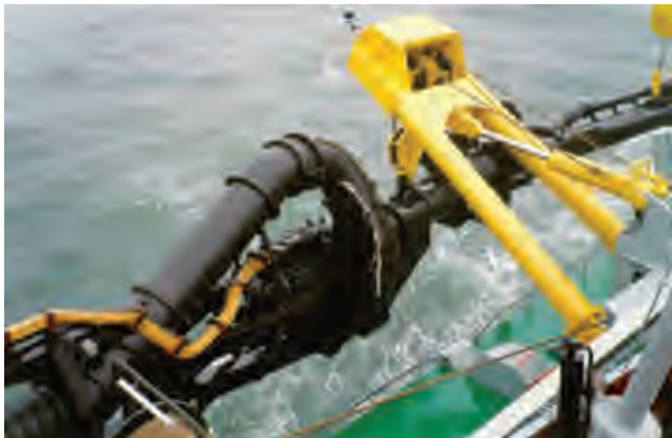
Figure A.14 Gantry for hoisting and lowering suction pipe on board a trailing suction hopper dredger.
