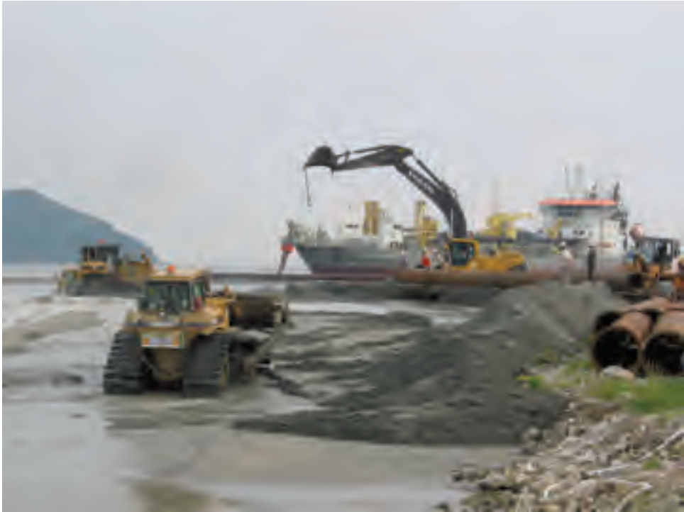
Figure 6.11 Construction of bunds above water level.
