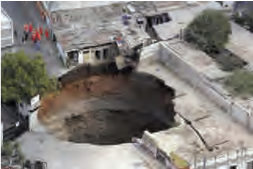
Figure 9.45 Massive sinkhole in Guatemala.
