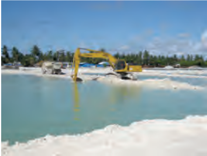
Figure 6.7 Truck dumping (end tipping) and profiling with excavators.
