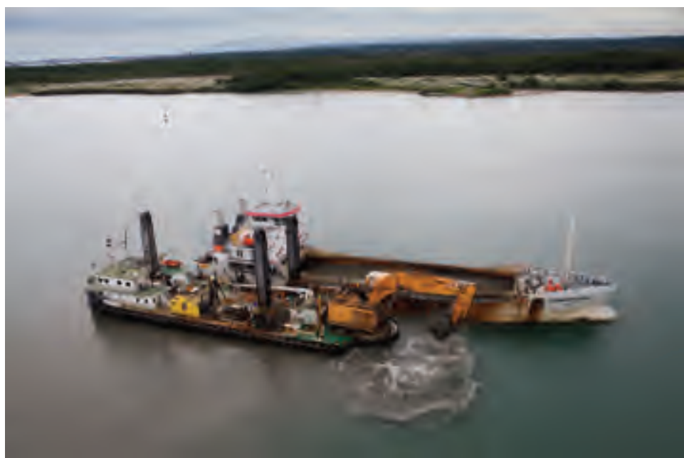
Figure 9.35 Backhoe: Dredging blasted basalt in the Panama Canal (bucket size = 11 m 3 ).
