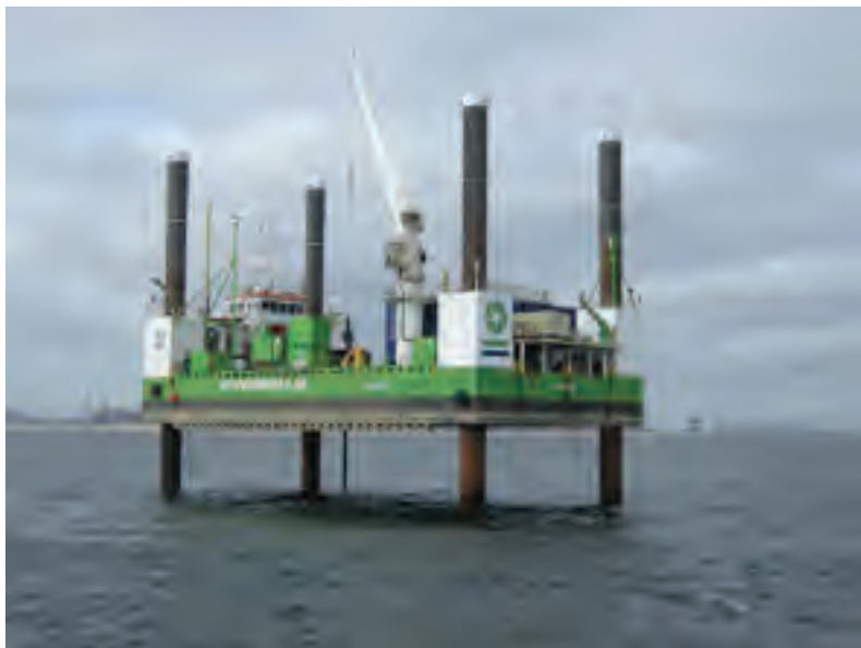
Figure B.10 Drilling from a jack-up platform.
