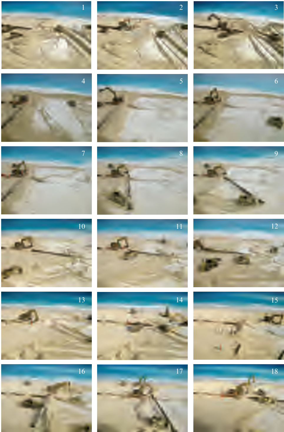
Figure 6.14 Typical work method beach nourishment (Canon beach reclamation).
