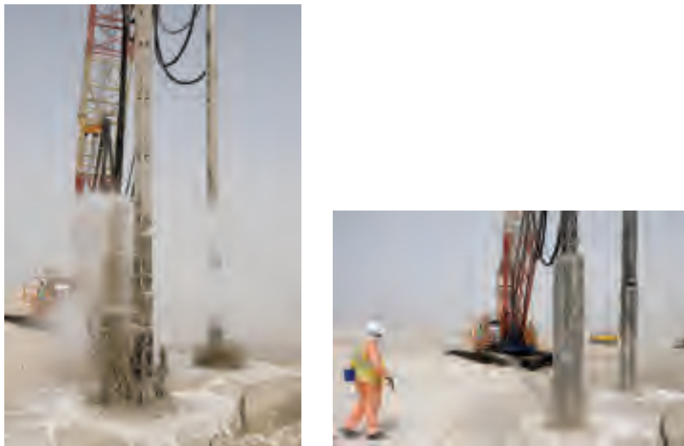
Figure 7.13 Crane mounted with tandem vibratory probes.
