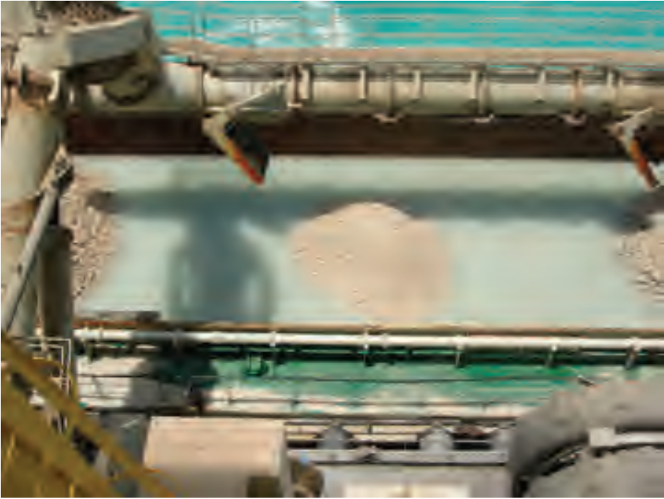
Figure 9.33 Barge loading with dredged rock.
