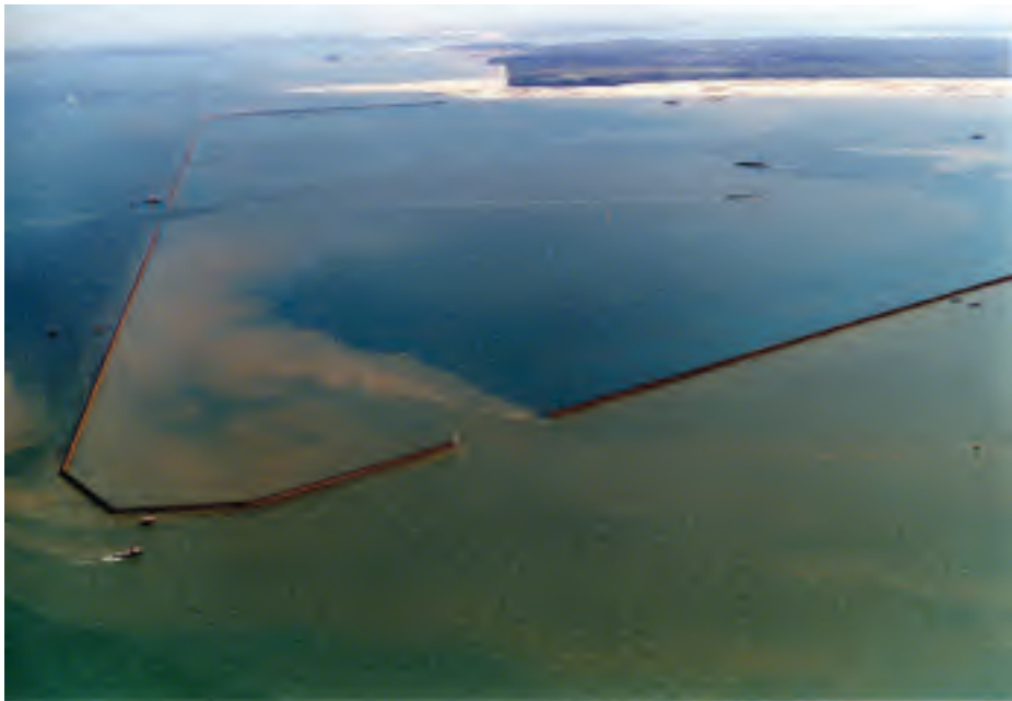
Figure 9.15 Construction of perimeter bund near Tekong island – Singapore.
