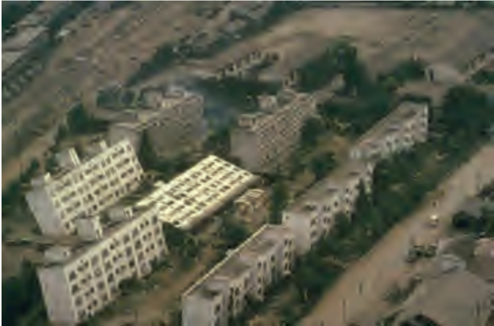
Figure 10.12 Liquefaction in a housing area, Nigata, Japan, 1964.
