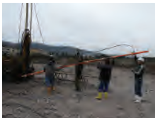
Figure B.47 Installation of extensometers in borehole.
