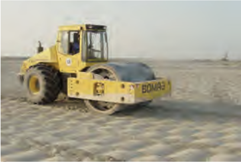
Figure 7.5 A polygonal drum compactor (after Mengé, 2007): Observe the impacted surface of the ground.
