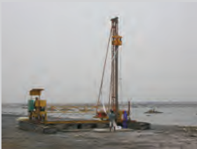
Figure 9.7 Installation of vertical drains using dual-hull amphibian equipment.
