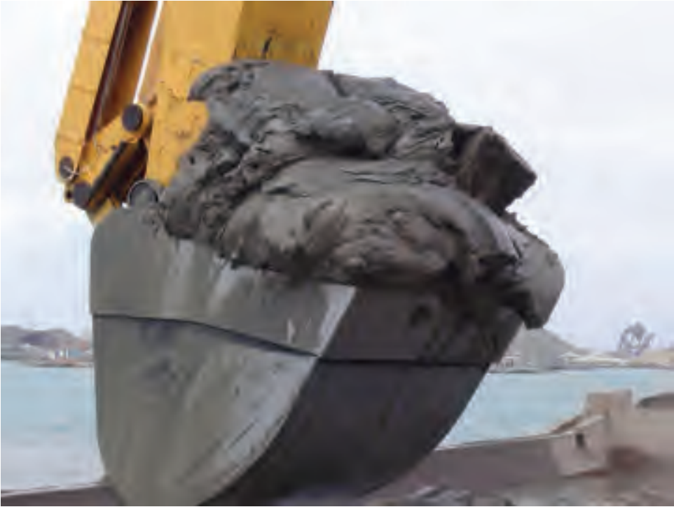
Figure 9.17 Dredging silt with a backhoe dredger.
