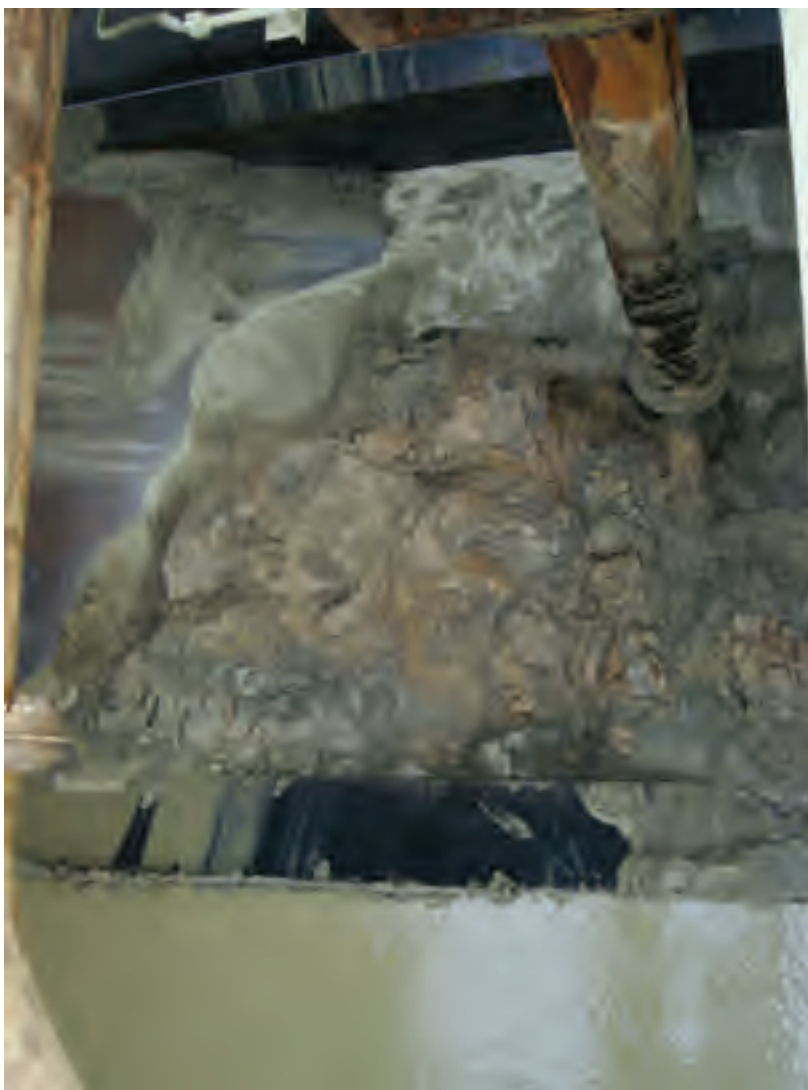
Figure 9.16 Sticky stiff clay inside a hopper – difficult to discharge.
