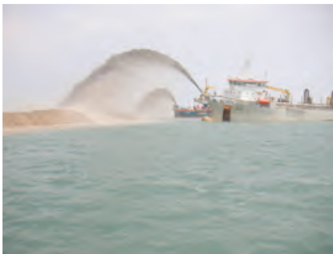
Figure 6.9 Bund construction using rainboring.
