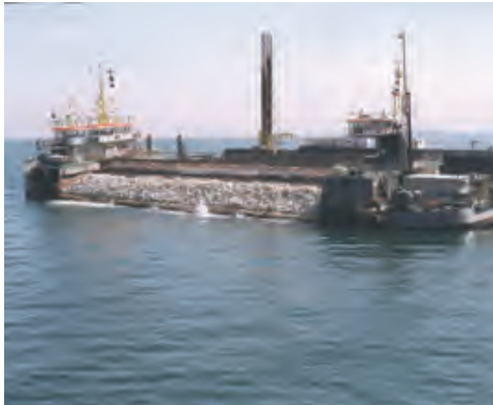
Figure 6.8 Side stone dumping vessel at work.
