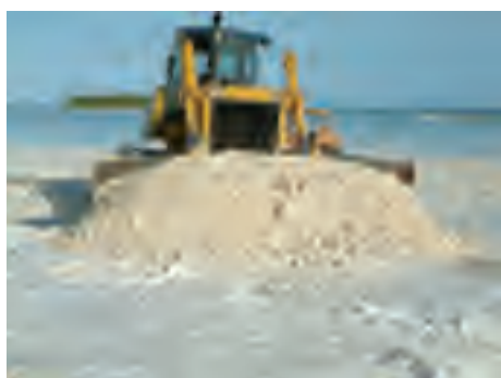
Figure 6.6 Rainbowing and subsequent shaping of the sand pancake.
