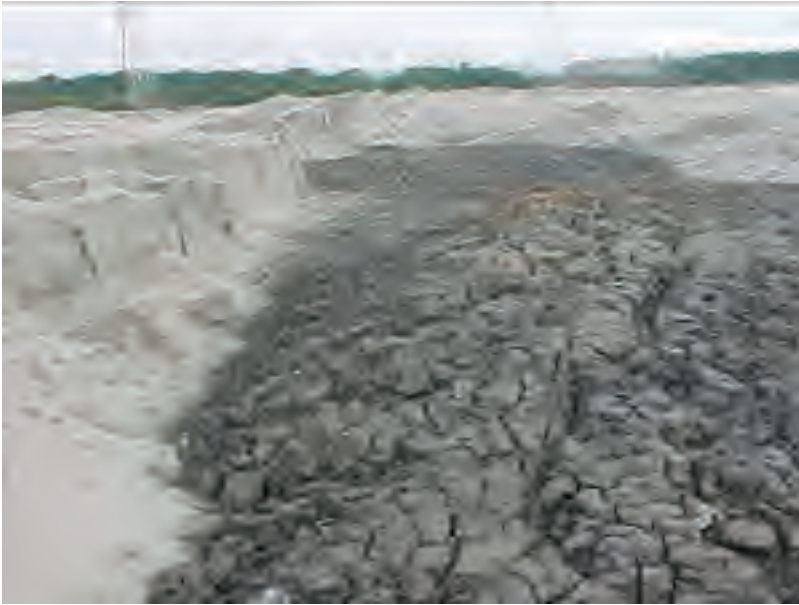
Figure 6.16 Mud wave on fill area.
