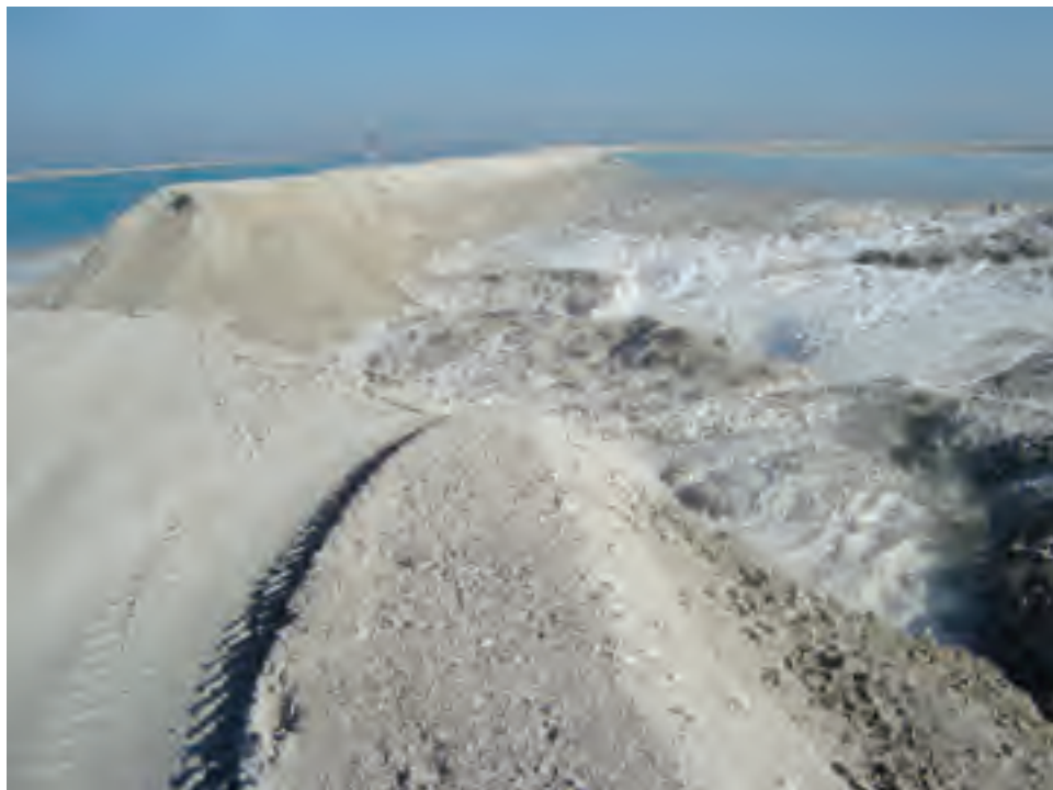
Figure 8.28 Failure of a hydraulic fill bund.
