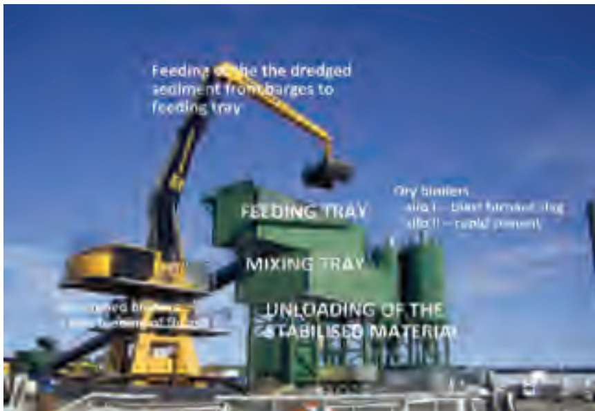
Figure 9.4 Process stabilisation – Turku project, Finland.
