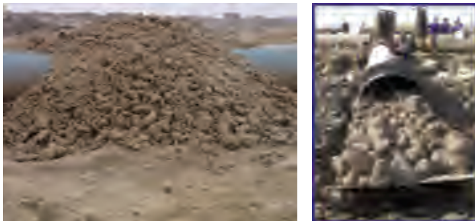
Figure 9.18 Formation of clay balls on the reclamation area.
