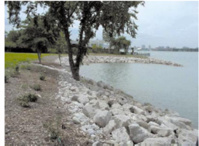
Figure 21 Goose Bay Park shoreline, after rehabilitation, is protected from erosion and enhanced for fish and wildlife habitat.
