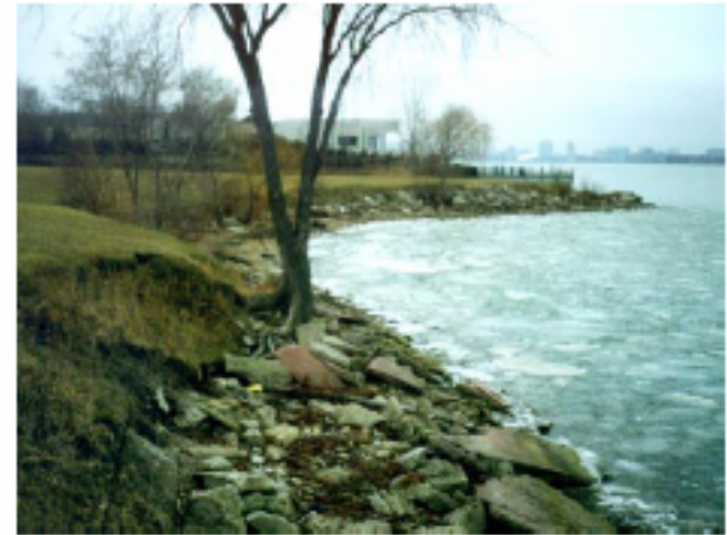
Figure 21 Goose Bay Park shoreline, after rehabilitation, is protected from erosion and enhanced for fish and wildlife habitat.
