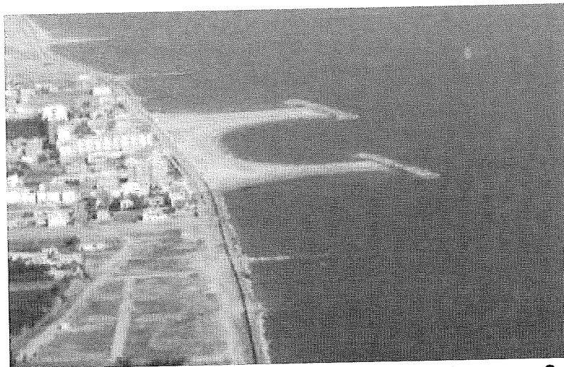
Figure 6-17 Tombolos behind two breakwaters at Almanzora, Spain
