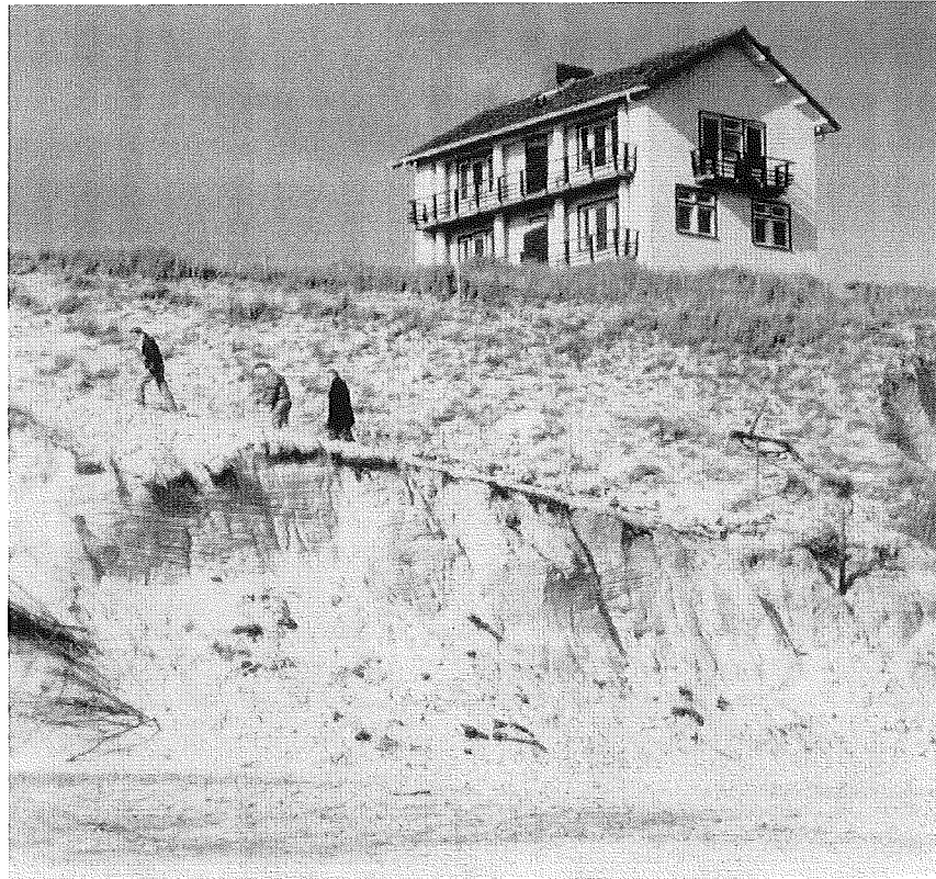
Figure 10-3 Damage because of dune erosion
