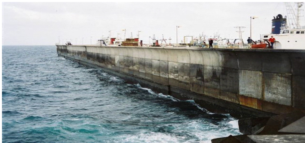
Fig. 16.17. An example of a modern, large vertical breakwater with wave return wall (left) and cross-section of an older seawall with recurve (right).
