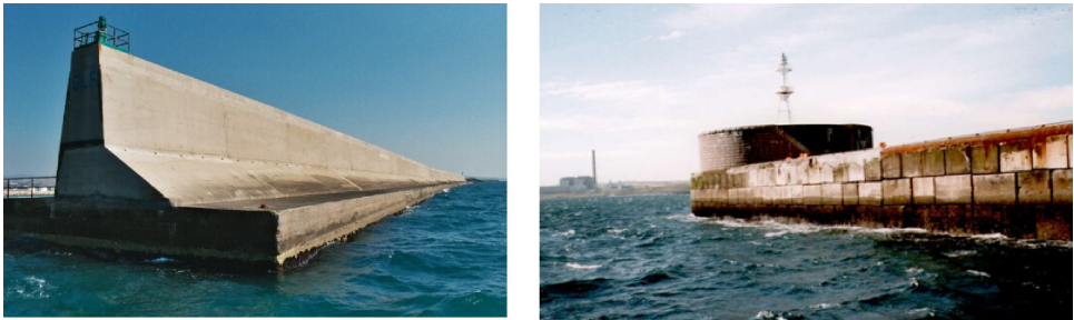
Fig. 16.1. Examples of vertical breakwaters: (left) modern concrete caisson and (right) older structure constructed from concrete blocks.
