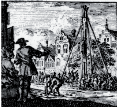
Figure 7.6 Dutch pile driving equipment (Huizinga 1985)
