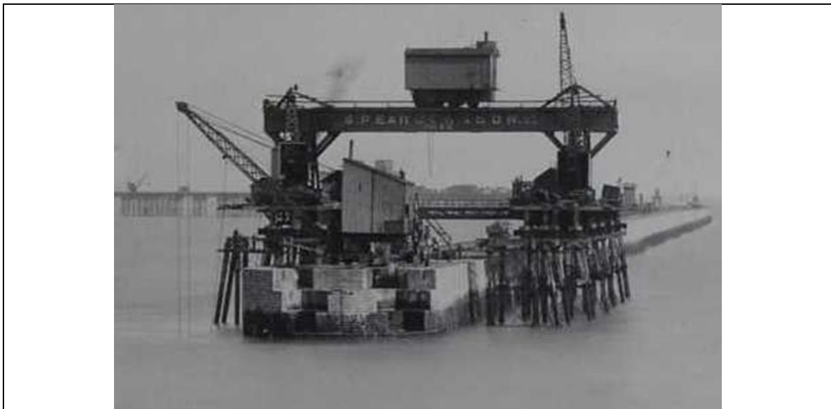
Figure 12 Goliath crane on staging (courtesy Dover Harbour Board)
