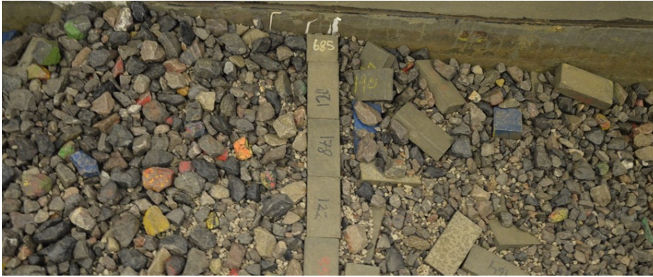
Figure 10: Post collapse view of Series 2, seaward side to right. Note the intact remnant of the wall toe.
