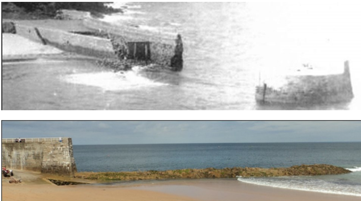
Figure 4: Greve du Lecq, Jersey: (top) after collapse in 1879; (bottom) recently, 2014
