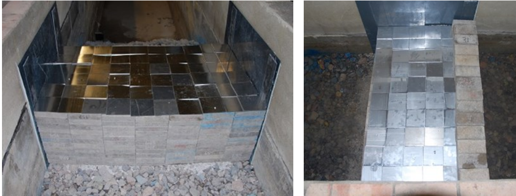
Figure 14: Test section for Series 5, showing crest slabs and parapet wall.
