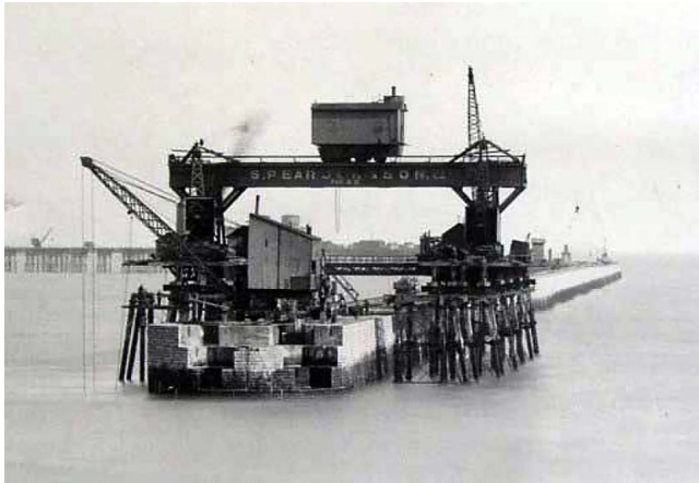
Figure 9. Goliath crane on staging (courtesy of Dover Harbour Board)
