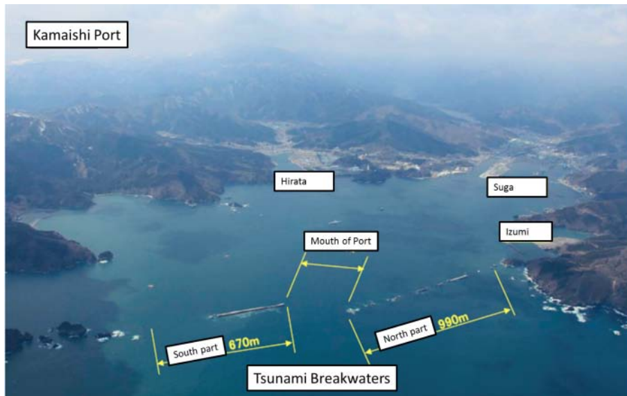
Photo 1. The Kamaishi Bay mouth breakwaters (taken by Tohoku Regional Bureau)
