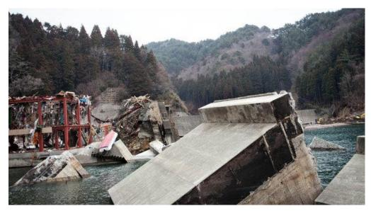
Figure 7: A section of the destroyed Kamaishi breakwater
