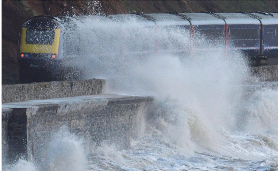
Figure 3.23: Wave overtopping onto a moving train, UK
