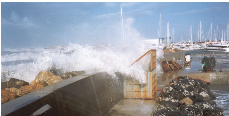
Figure 3.18 Measuring real wave overtopping during CLASH at Ostia, Italy.
