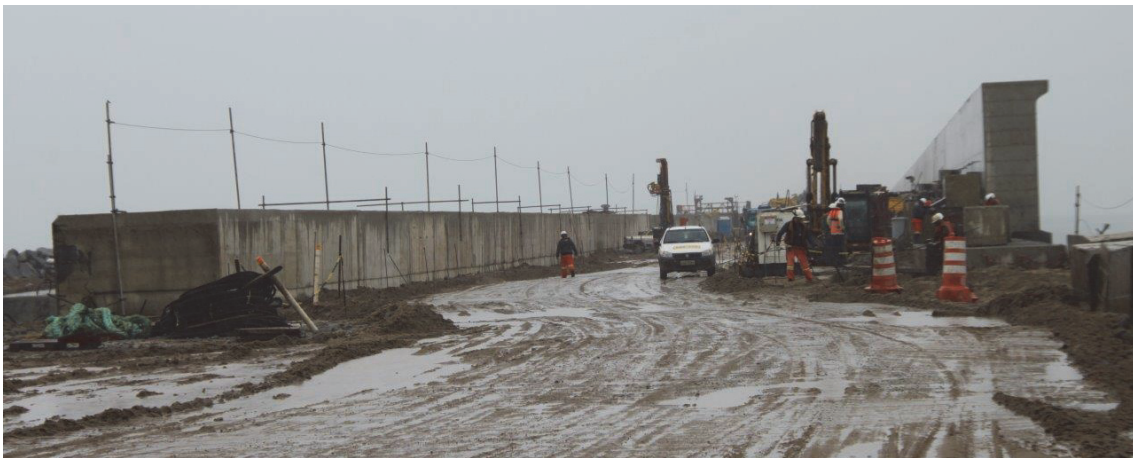
Figure 1.7: A relatively small bull nose on the crest wall of a large caisson. The caisson under construction, Açú, Brasil, is 25 m wide and the crest level is 10 m above sea level
