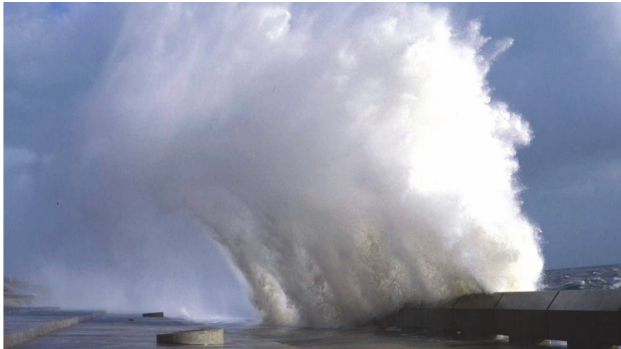
Figure 3.17 Severe wave overtopping at Samphire Hoe, UK.
