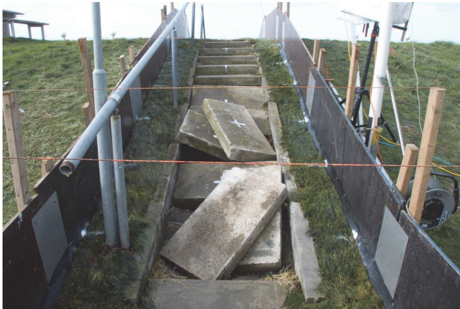
Figure 4.41 Testing a stair case with the new Wave Run-up Simulator in 2014
