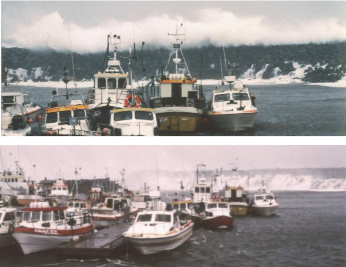
Figure 6.15: Rear side of the Bakkafjordur breakwater during a storm in 25 October 1995, overtopping over the crest and through the crest. Courtesy S. Sigurdarson
