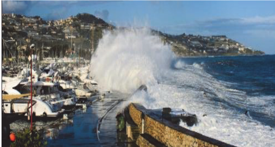
Figure 3.12: Wave overtopping at the marina of San Remo, Italy, damaging small boats
