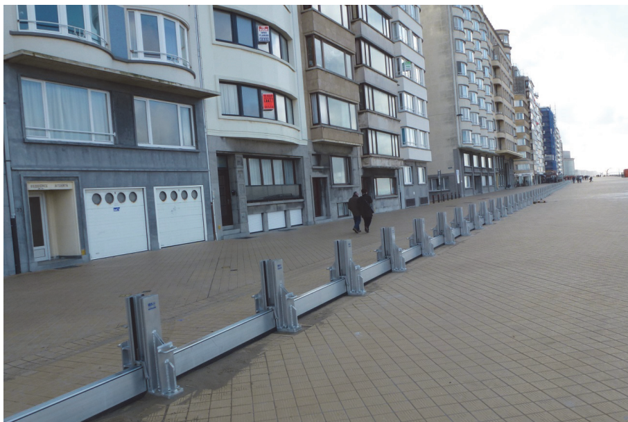
Figure 3.13: Apartments on the boulevard at Oostende, Belgium, protected by a movable storm wall to reduce impacts by overtopping waves
