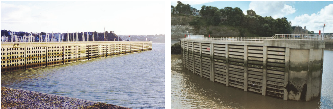
Figure 7.24: Examples of perforated caissons, left Caen, France and right Cardiff Barrage, UK
