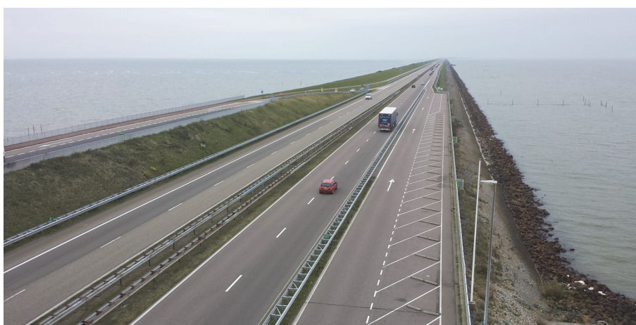
Figure 3.22: The highway on the Afsluitdijk, the Netherlands, with the Wadden Sea and the sea defence on the left side and the fresh water lake, the IJsselmeer, on the right side
