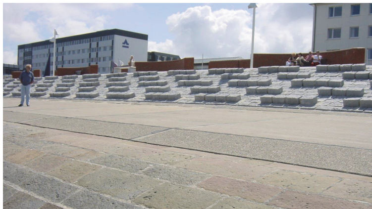
Figure 5.26: Example of battens or ribs in reality
