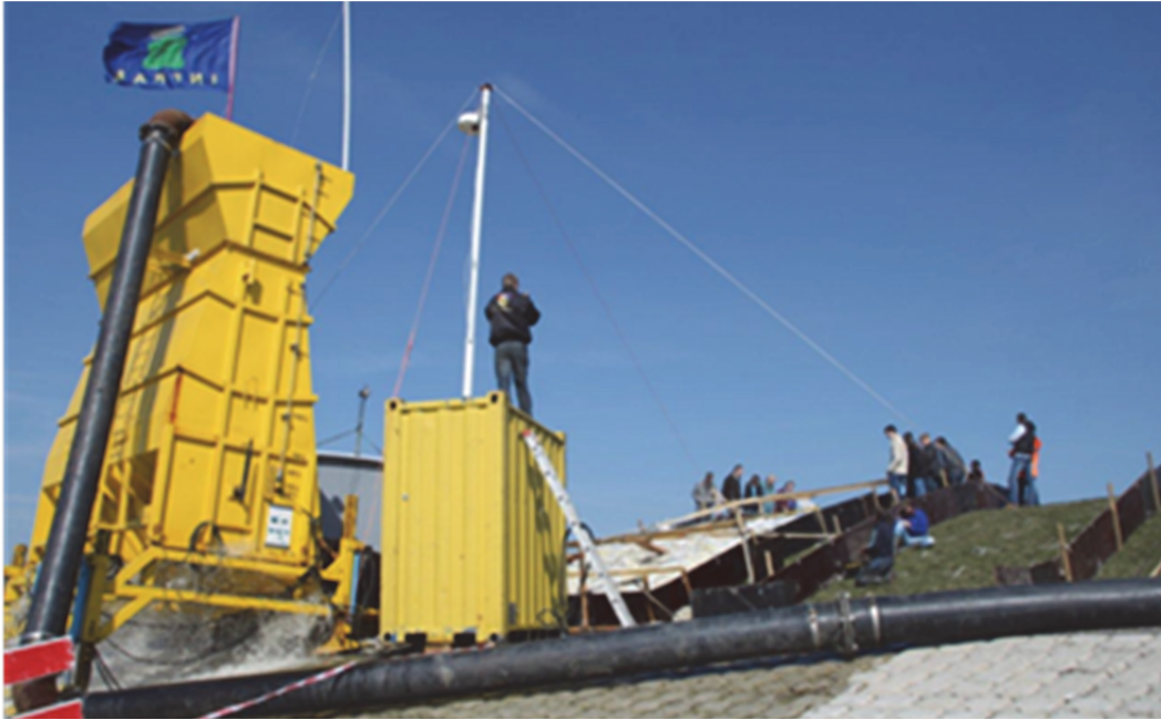
Figure 4.38 Pilot wave run-up test at Tholen, using the existing Wave Overtopping Simulator
