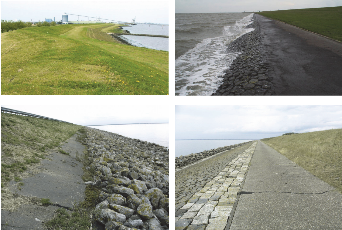
Figure 5.1: Examples of coastal dikes, levees and seawalls. Delfzijl, NL; Busum, DE; Houtribdijk, NL; Rotterdamse Hoek, NL
