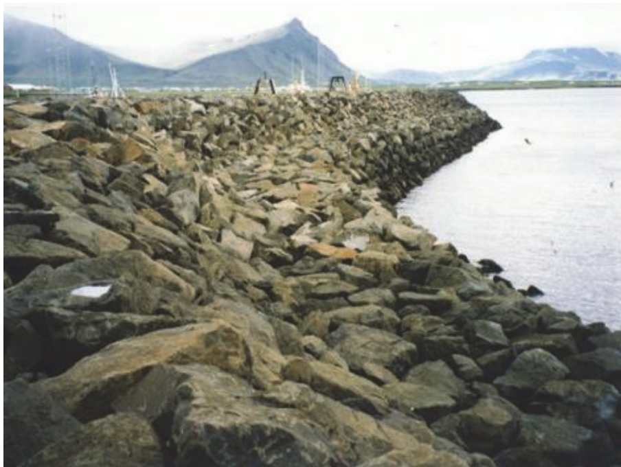
Figure 6.10 Icelandic-type berm breakwater
