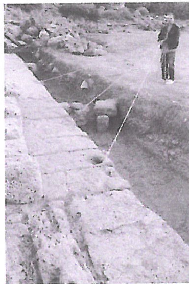
Figure 4 Part of quay with binding holes and mooring stones (Hadjidaki and Stefanakis, 2004: 115).
