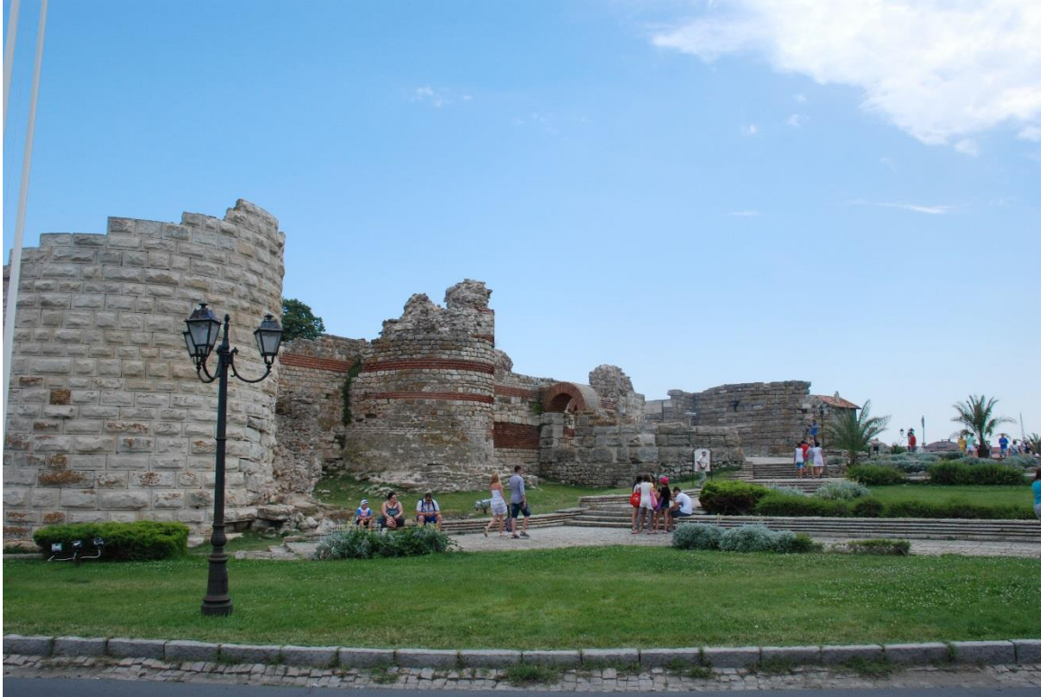
Fig.3. Bulgaria, Nessebar. General view of the walls
