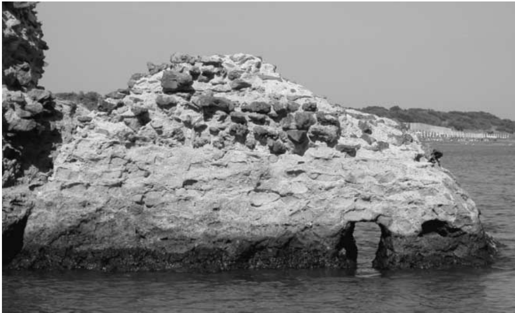
Figure 4. Cosa: Pier 2, side view from west.
