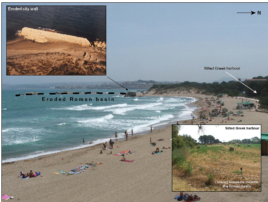
Fig. 21. Ampurias' Roman harbour. Exposed wave conditions coupled with avulsion of the river Fluvia to the north of the settlement have led to a fall in sediment supply and a gradual erosion of the harbour infrastructure during the past two millennia. The ancient Greek harbour had to be abandoned due to silting up of the basin (photographs: Marriner).
